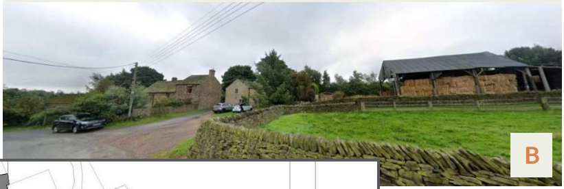
Access off High Lane to Willow House
