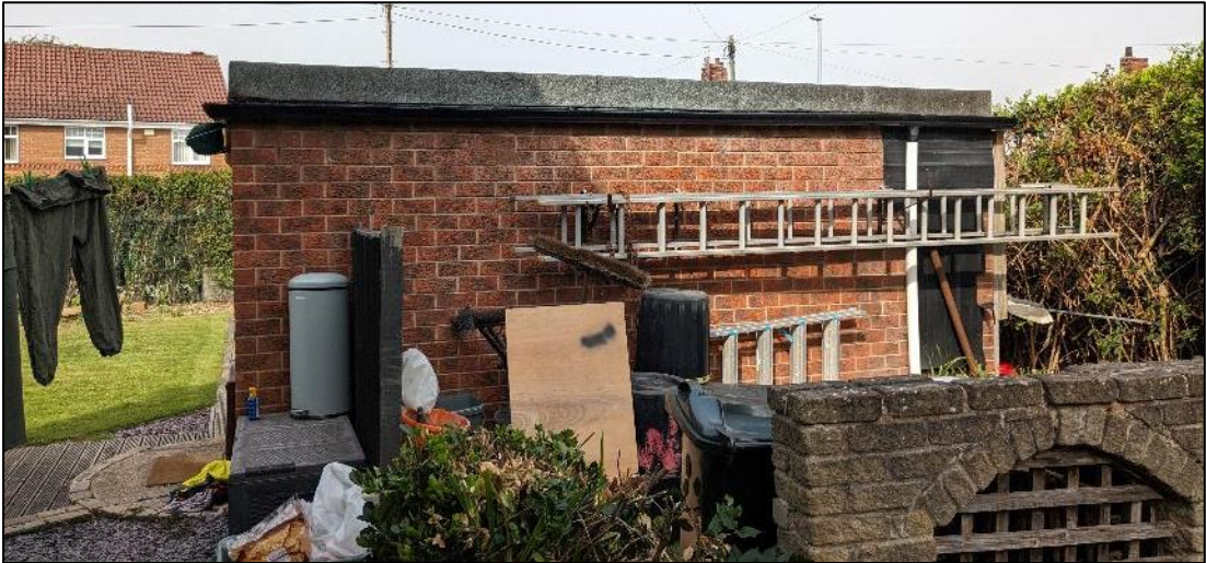
Plate 6. Southwest elevation of outbuilding
