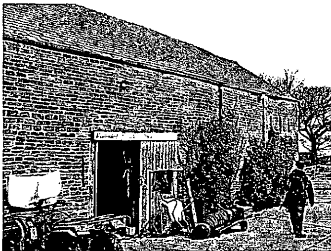
Picture shows existing store building.
