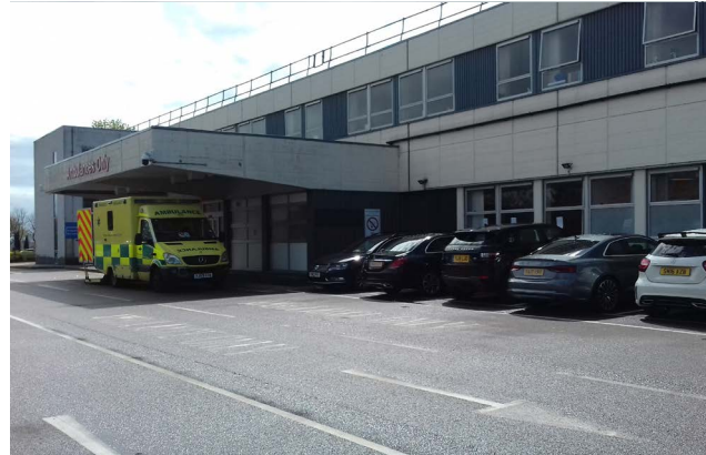
Access lanes for ambulances and projecting canopies
