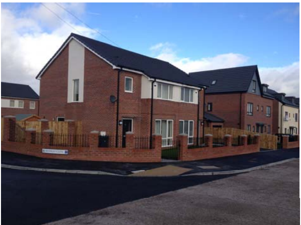
New housing on the north side Langsett Road
