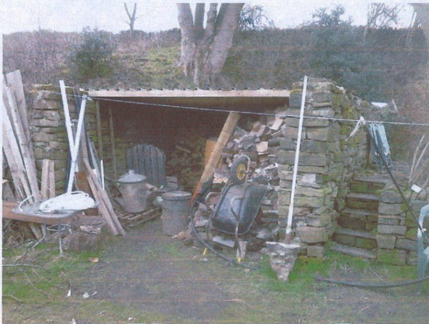
Photograph 3 - Building to be extended
