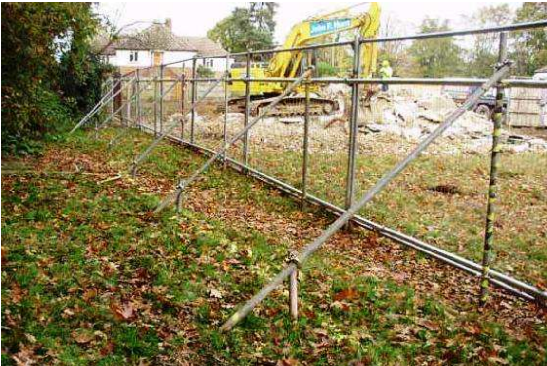
Figure 2: Photo of Fencing to BS 5837:2012
