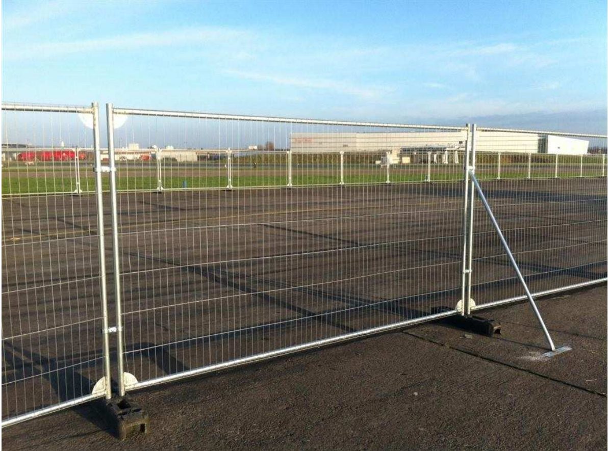
Figure 6: Secured 'Heras' type fencing with stabilizing system and anti-tamper couplers
