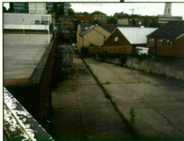
Figure 4: View of the goods delivery area from the Pitt Street footbridge.
