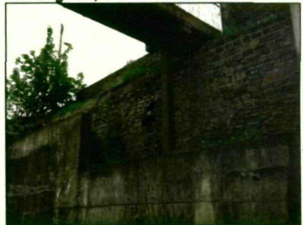
Figure 12: The stone-built section of the retaining wall, with Pitt Street above.
