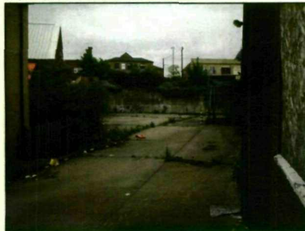
Figure 5: View of the goods delivery area from the Peel Street access.
