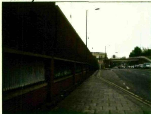
Figure 3: View of the south elevation on West Way.
