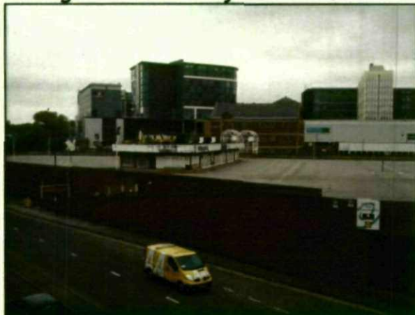
Figure 1: View of the roof top car park looking across West Way from Pitt Street.
