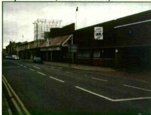
Figure 2: The Peel Street shop frontage and car park access (north elevation).
