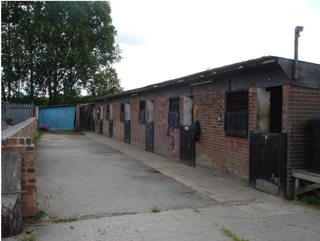
05. Building D Stables – North Elevation
