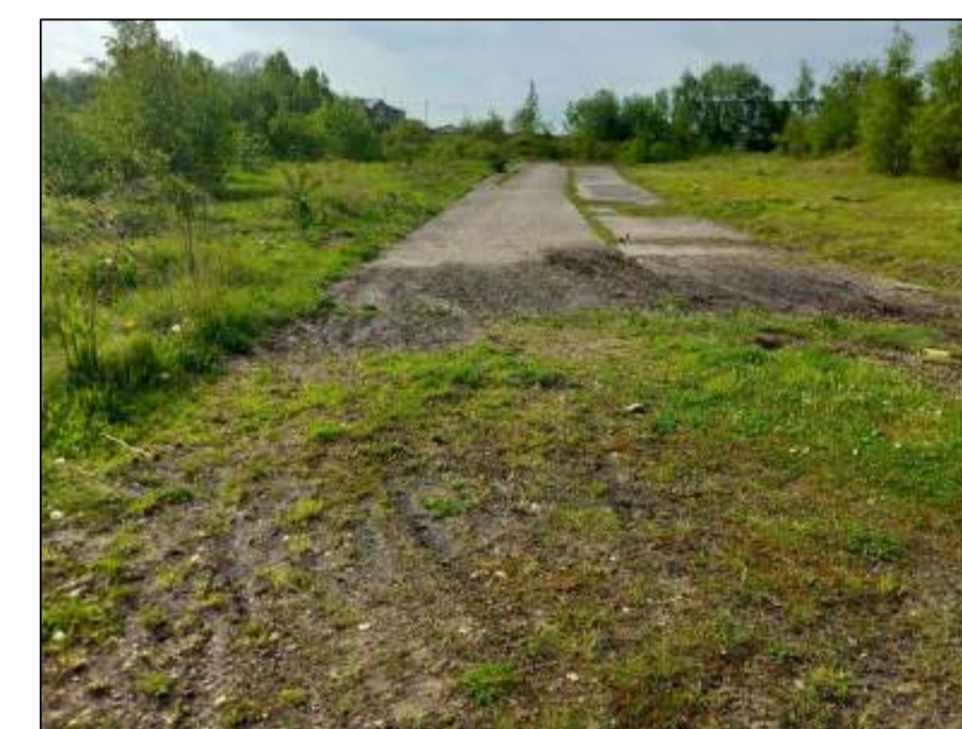
8. View south showing concrete slabs.
