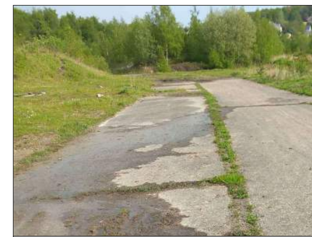
7. Concrete slabs and ecological exclusion area.
