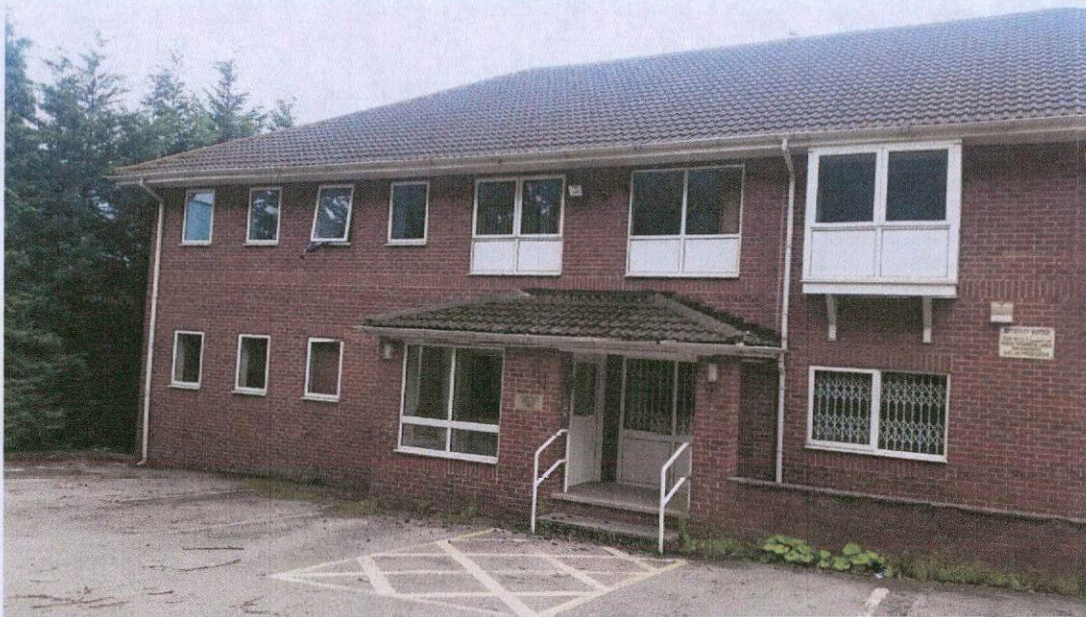
Picture 1: Compass House. This measurement location is labelled ML1 at the front of the building.
