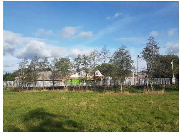
Photo 2: T3 to T17 from west
