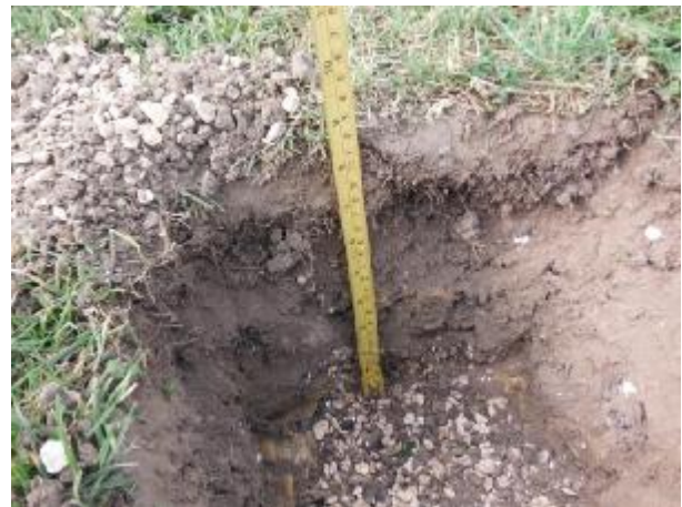
Fig 4: Drain excavated
