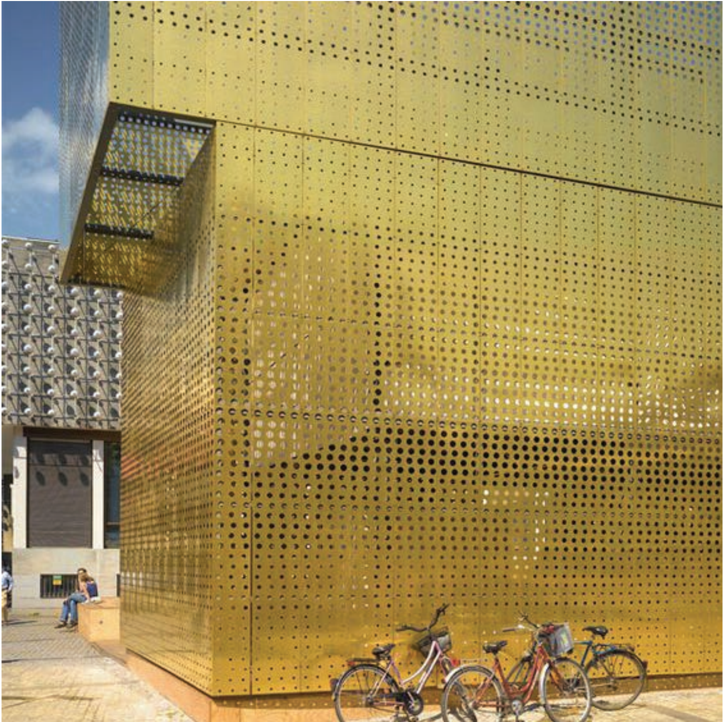
Perforated metal screen - bicycle storage beneath bridge deck
