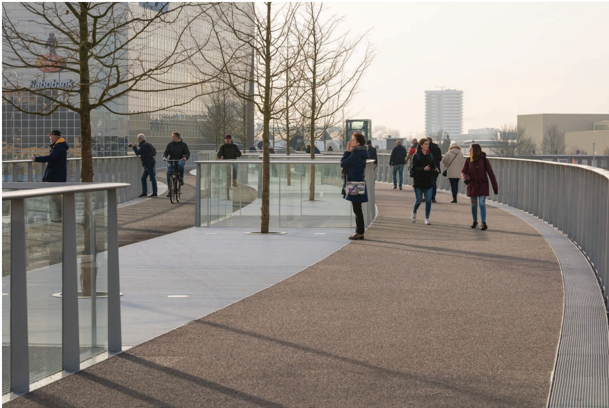
Resin finish to the bridge deck
