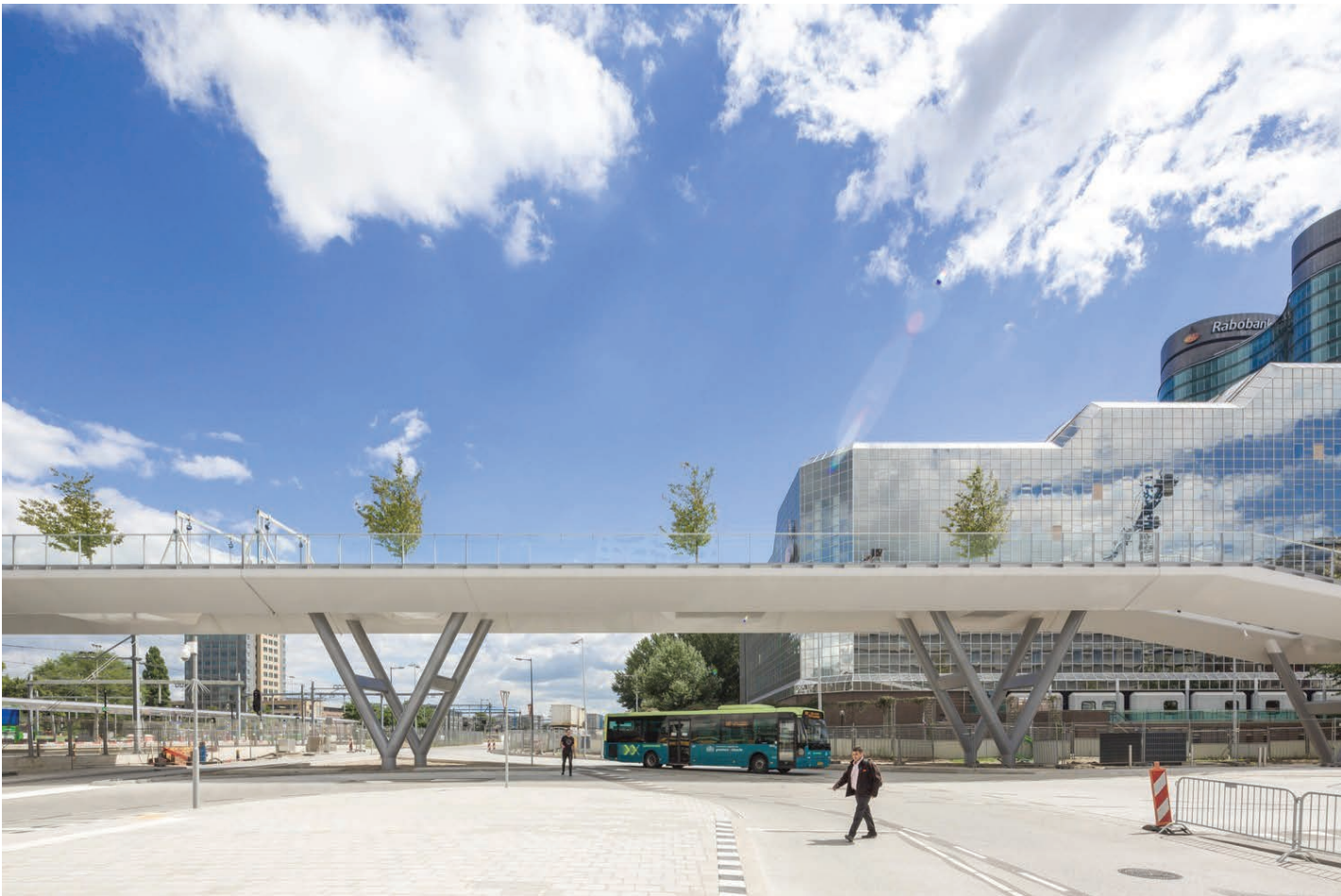
White painted steel pedestrian bridge, Utrecht
