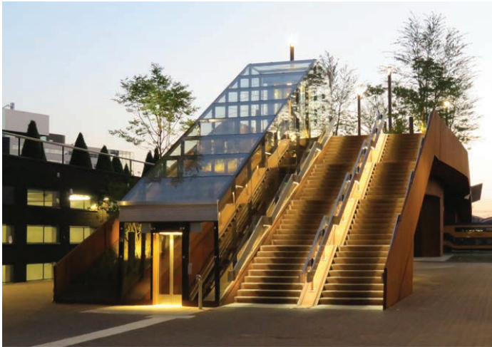
Strip LED's to handrails
