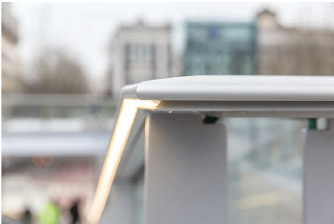
Strip LED's to handrails
