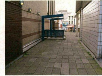
8. Access ginnel (ground floor)
