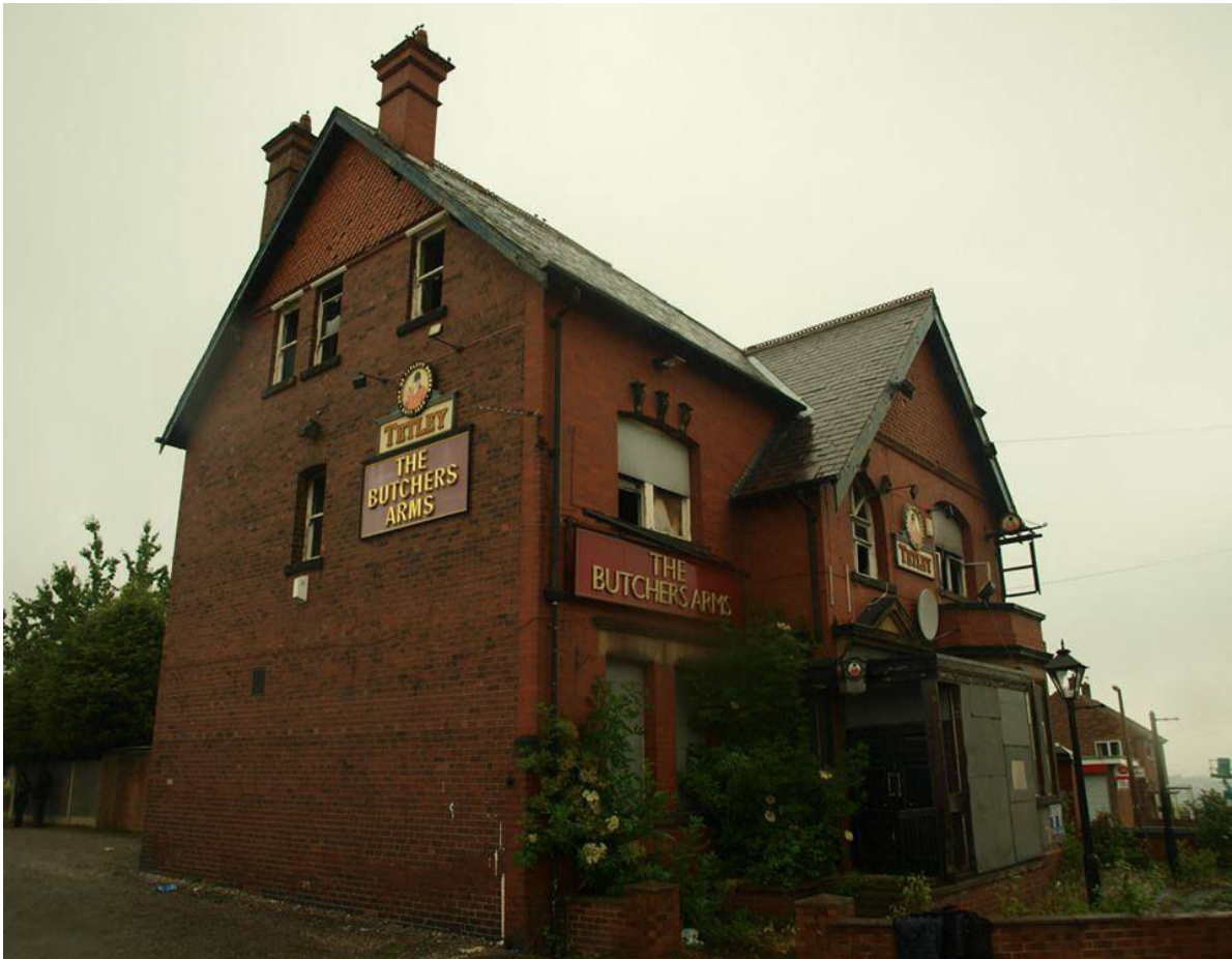
Above: Previous Public House prior to demolition
