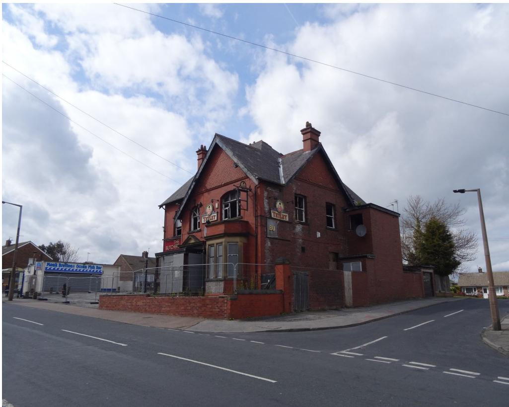
Above: Days before demolition – looking North from High Street
