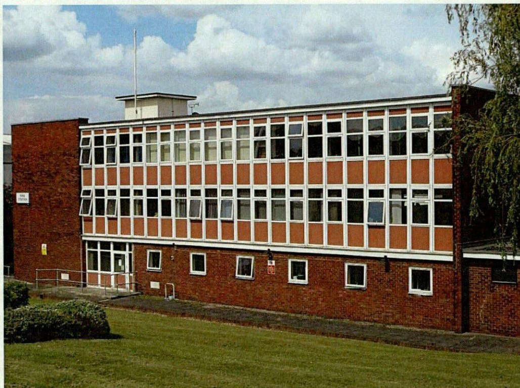
Plate 5: Fire station, south-west elevation
