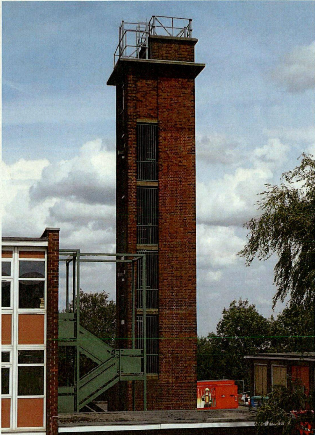
Plate 7: Drill tower, looking north-east
