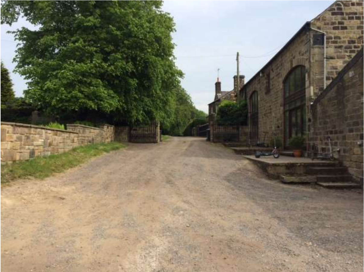
Site Access - Viewing Eastwards adjacent to the existing dwellings
