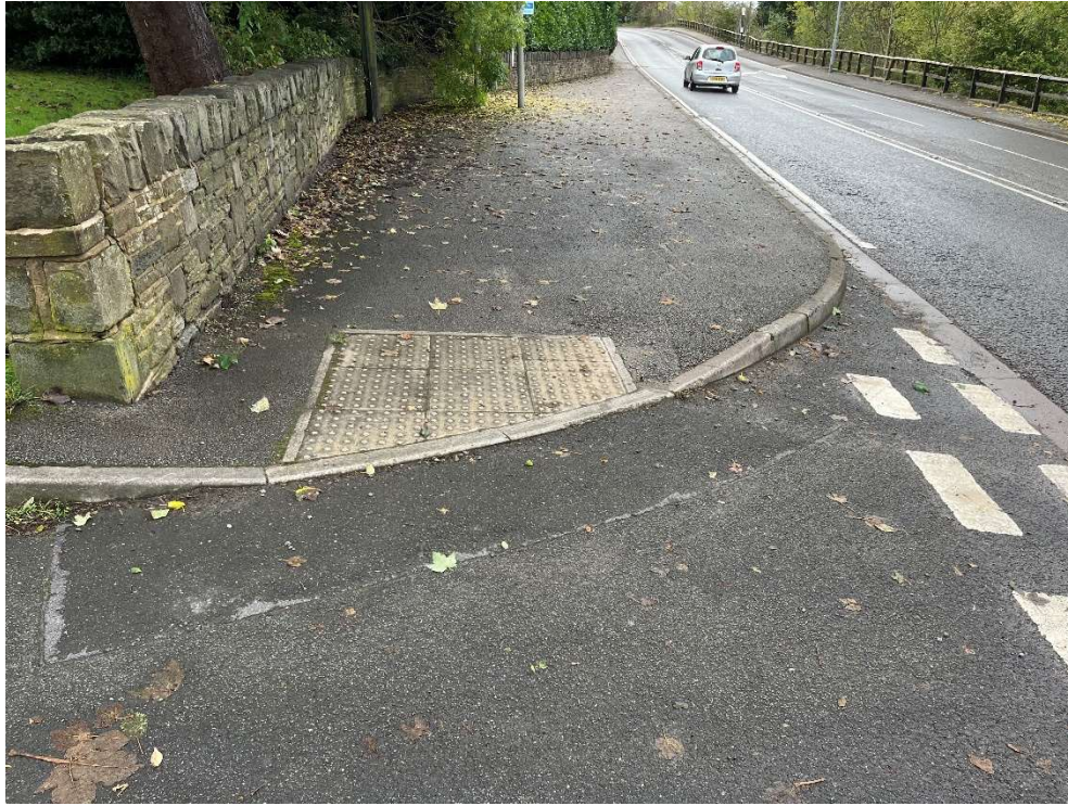
Balk Farm Court kerb right side radii line at junction with Sheffield Road
