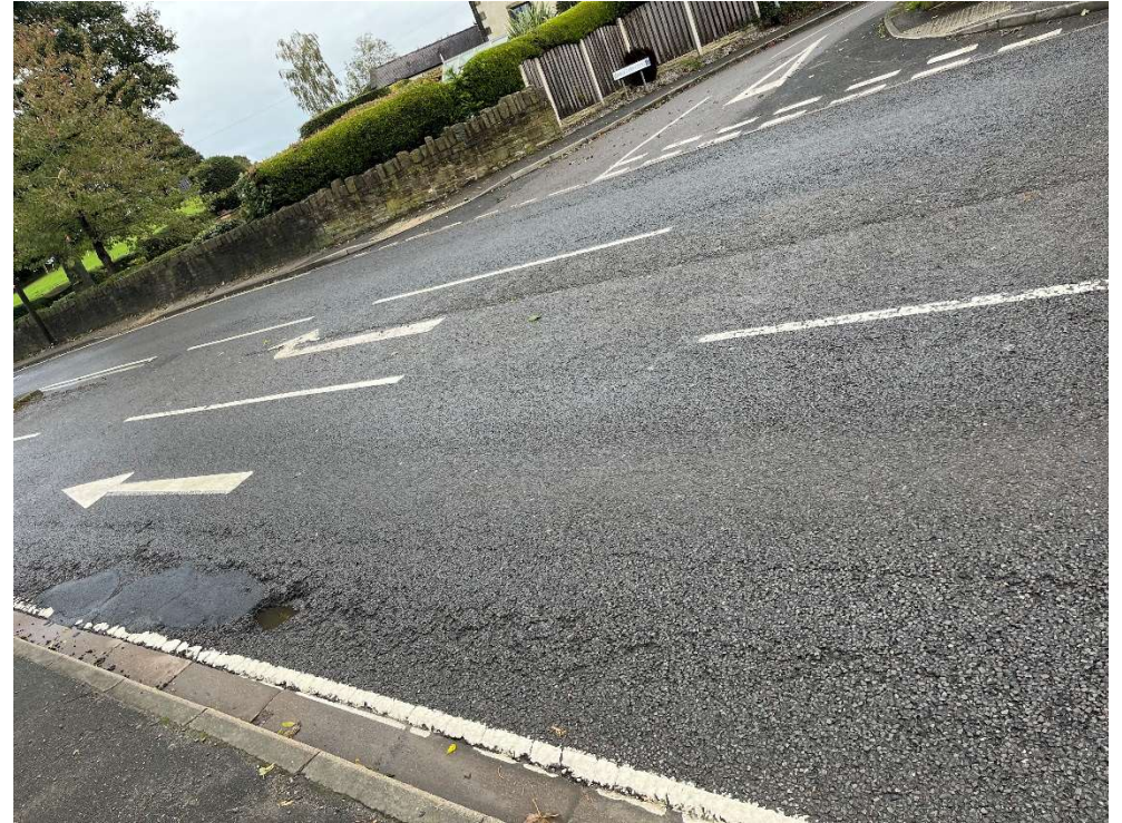
Sheffield Road repairs opposite Balk Farm Court junction
