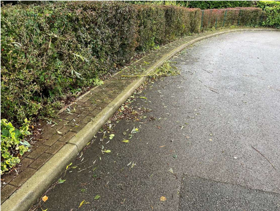
Balk Farm Court kerb right side kerb line above site entrance
