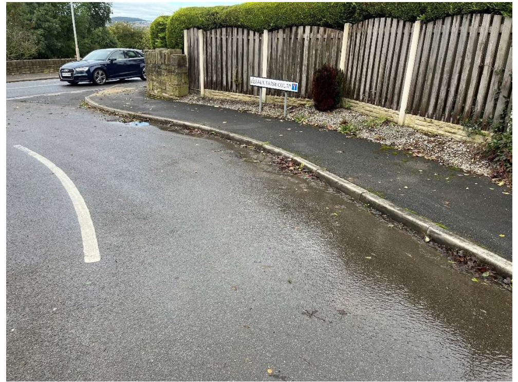
Balk Farm Court left side kerb at junction with Sheffield Road
