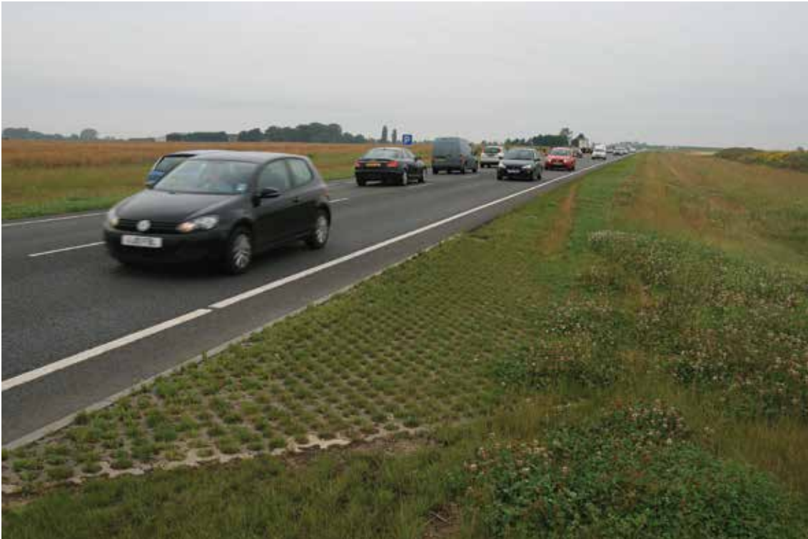
Figure 9.3 Swale and wetland systems with reinforced grass used in less trafficked areas such as laybys and field access points, A16, Lincolnshire (courtesy EPG Limited)
