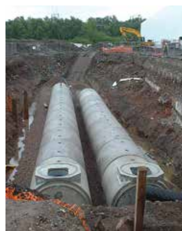
Figure 11.11 Rainwater harvesting storage tanks during construction (courtesy British Precast)
