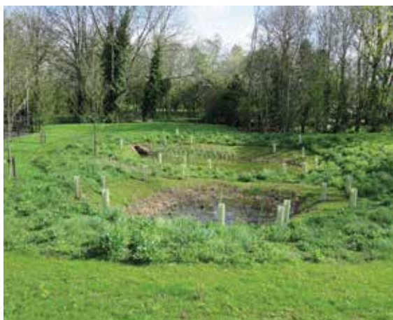
Figure 6.8 Infiltration basin with wildflower turf and grass seeding, Victoria Park Health Centre, Leicester (courtesy DSA Environment and Design)
