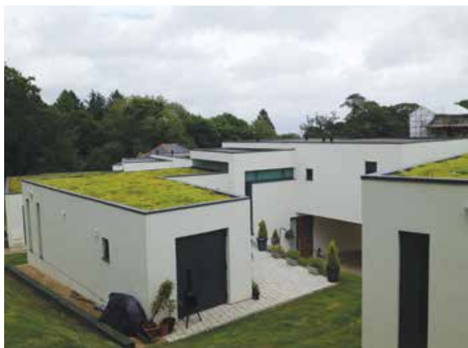
Figure 12.5 Domestic green roofing, Swansea (courtesy Sky Garden)
