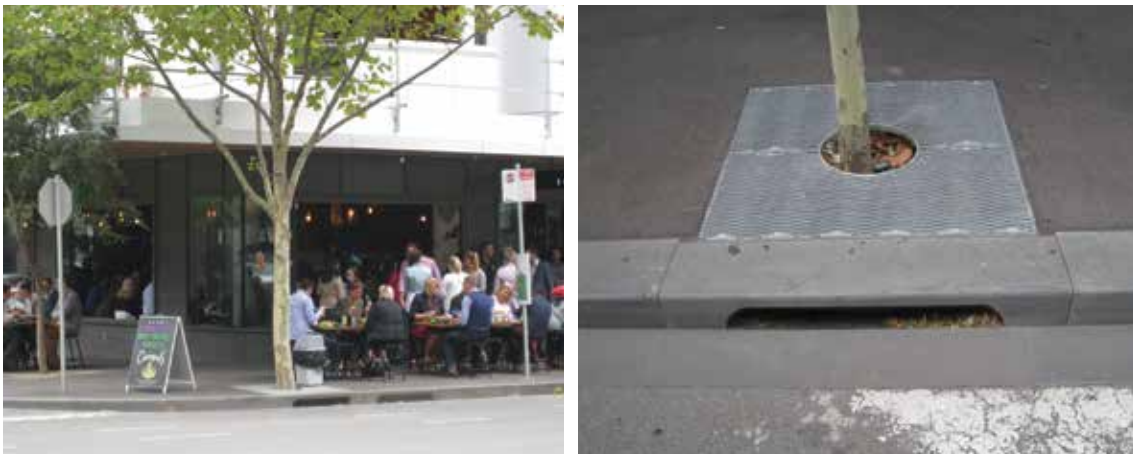
Figure 19.6 Tree pit in Bourke Street, Melbourne
