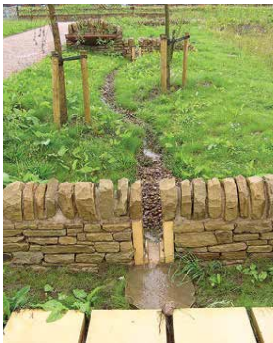
Figure 17.12 Check dam wall using local materials, Sheffield (courtesy Sheffield City Council)
