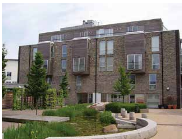
Figure 23.16 Geometric design of pond in an urban area, Malmö, Sweden (courtesy Illman Young)
