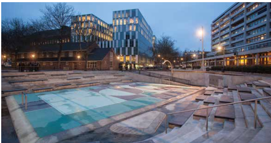
Figure 22.5 Example of urban hard surfaced off-line detention basin with geometric design to enhance amenity use, Rotterdam, the Netherlands (courtesy palleash+azarfane)
