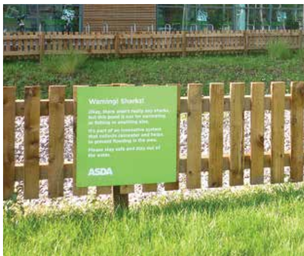
Figure 5.14 Signage and toddler-proof fencing at a supermarket site (courtesy ACO Limited)
