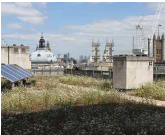
Green roof (courtesy Green Roof Consultancy)
