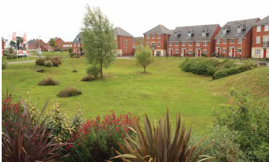
Figure 22.1 Detention basin with landscape design providing attractive amenity space, Hamilton, Leicester
