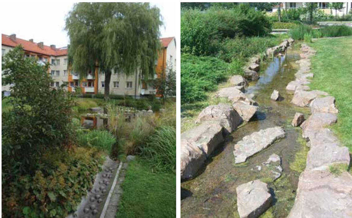
Figure 23.12 Energy dissipating inlet channels for ponds, Augustenborg, Sweden (courtesy Graham Fairhurst and Illman Young)
