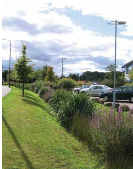
Figure 17.11 Linear wet swale, Junction 4 M8, West Lothian
