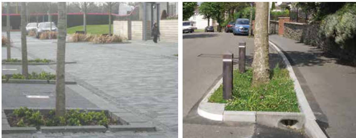
Figure 19.16 Examples of inlets to allow surface water runoff to infiltrate into tree pits (courtesy Anne Jaluzot and Dŵr Cymru Welsh Water)
