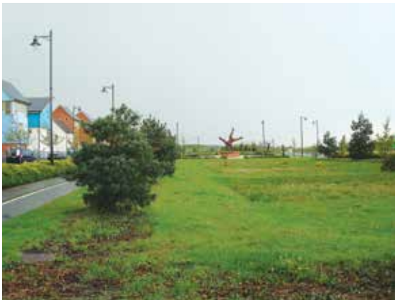
Figure 13.6 Large infiltration basins, Ipswich (courtesy Graham Fairhurst)
