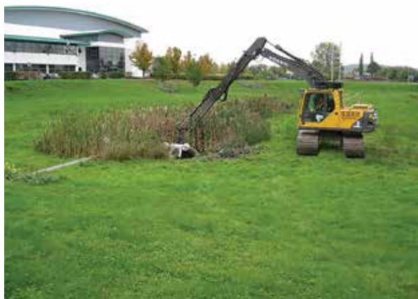
Figure 32.2 De-silting (courtesy Bedford Group of Drainage Boards)
