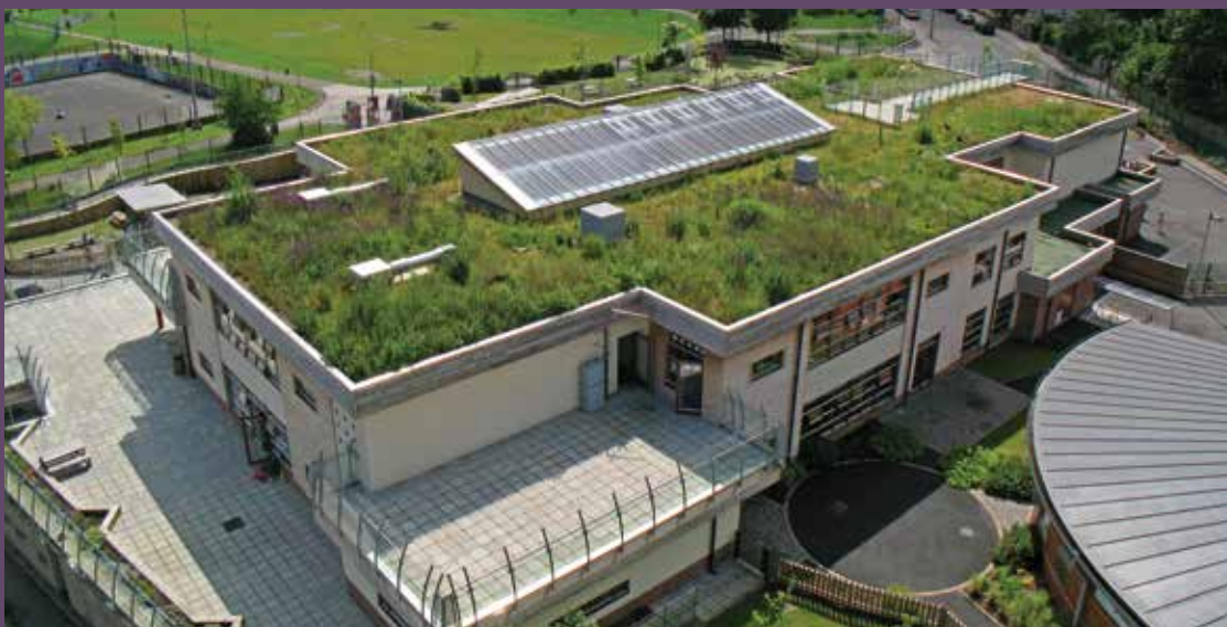
Figure 12.13 Sharrow School green roof (courtesy The Green Roof Centre)
