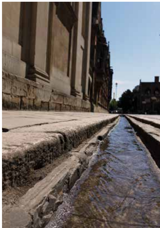
Figure 10.18 Roadside rills, Cambridge (courtesy Cambridgeshire County Council)
