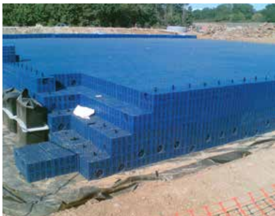
Figure 21.2 Structural frame being constructed (courtesy EPG Limited)
