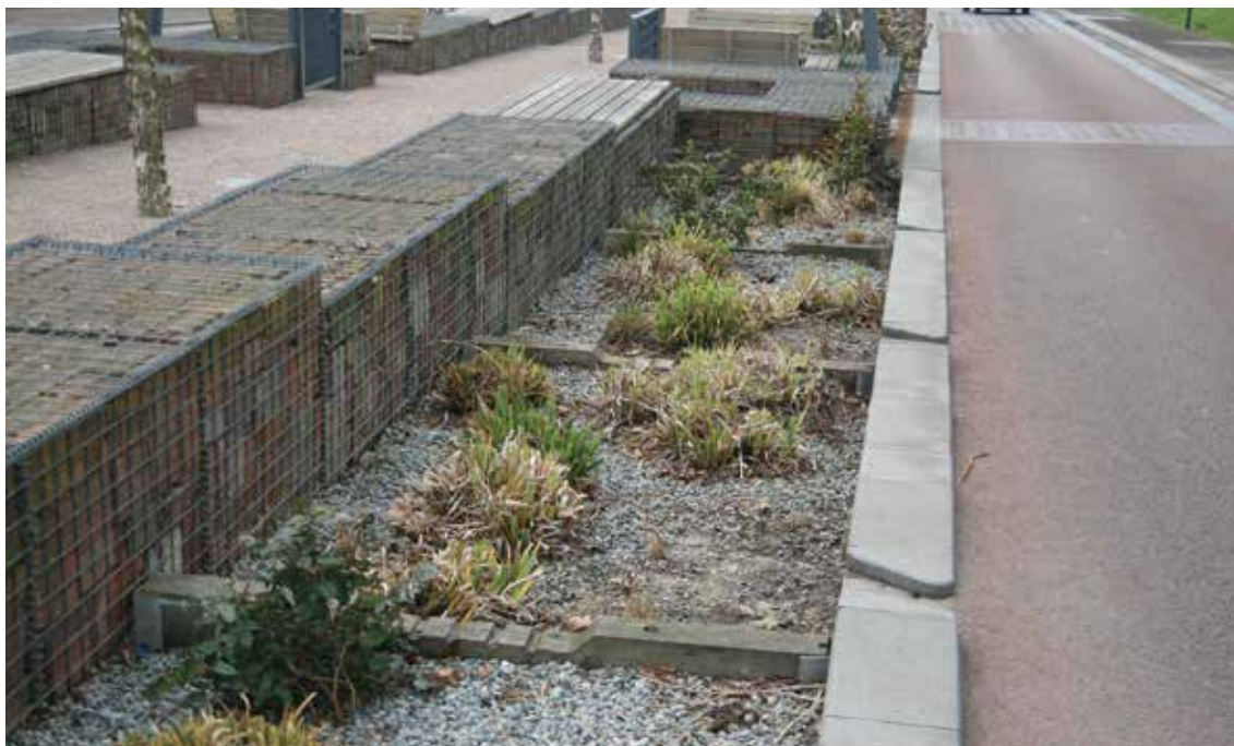
Figure 10.13 Rain garden with weirs to control flows on sloping site in Ashford, Kent (courtesy EPG Limited)
