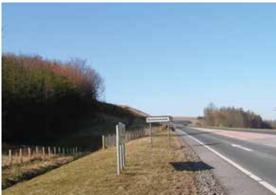
Figure 9.6 Filter drain, A7, Dumfries and Galloway (courtesy Hydro International)
