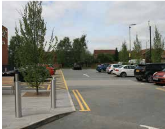
Figure 20.7 Retail development car park with porous concrete, High Wycombe (courtesy EPG Limited)
