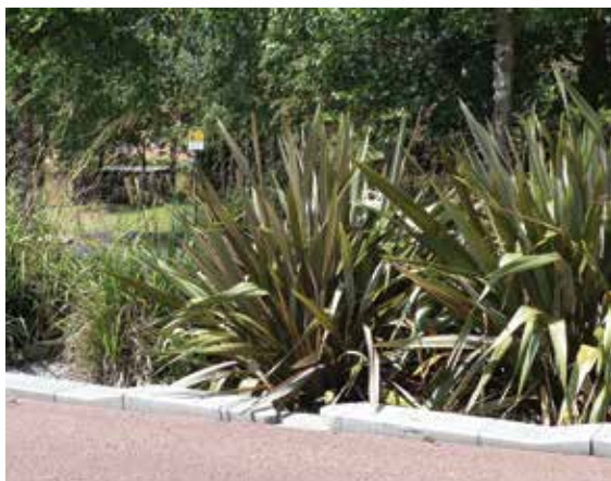
Bioretention system (courtesy Essex County Council)
