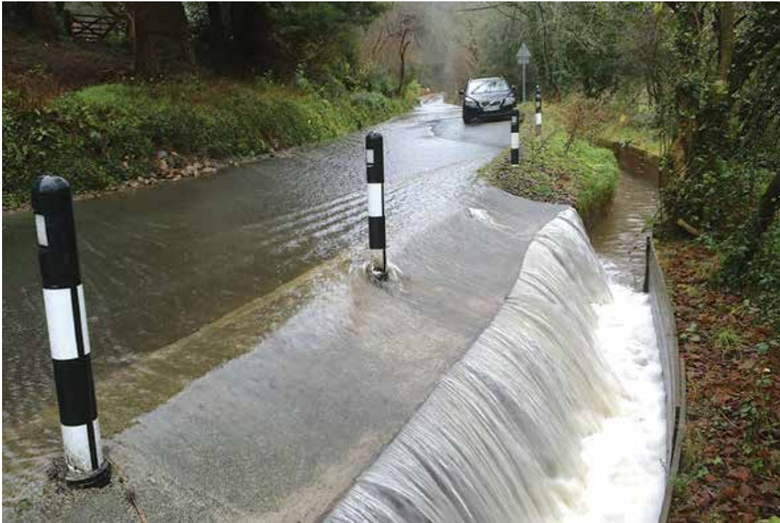
Figure 9.19 Highway acting as a flood pathway in an exceedance event (courtesy Simon Jeffrey)
