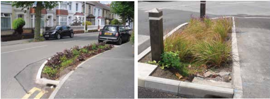
Figure 5.4 Examples of bioretention systems providing traffic calming measures, Llanelli (courtesy Dŵr Cymru Welsh Water)
