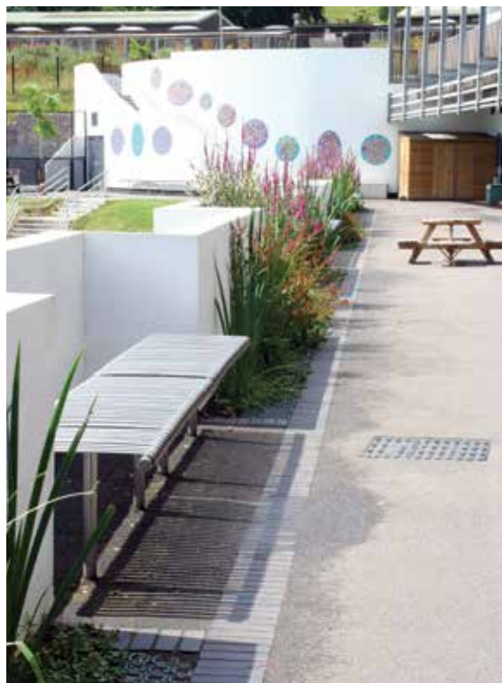
Figure 16.4 Filter drain with planting, Exwick, Devon (courtesy Robert Bray Associates)
