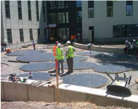
Figure 20.6 Construction of pavement using resin bound post consumer recycled glass aggregate (courtesy Filterpave Limited)
