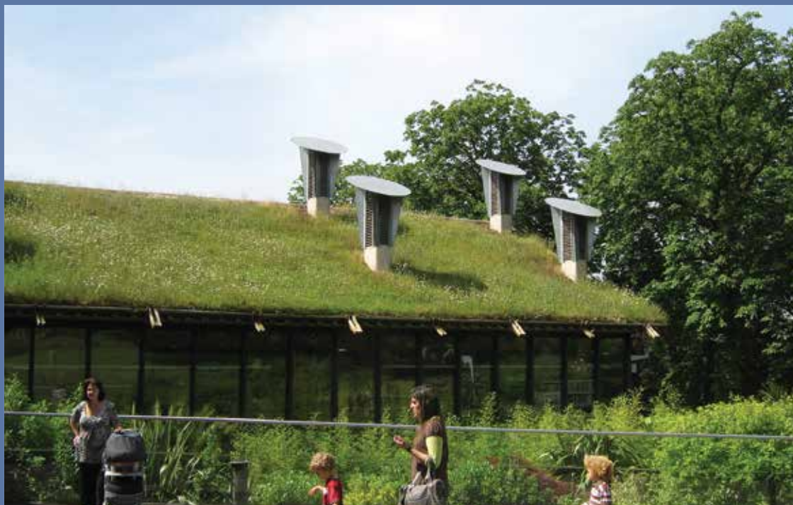
Figure 6.3 Green roof at Horniman Museum, London (courtesy Gary Grant)
