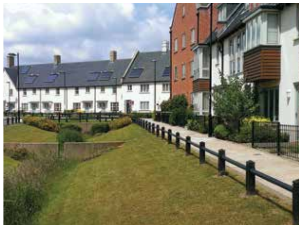
Figure 17.8 Dry swale with overlying flow control, Upton, Northamptonshire (courtesy Peterborough City Council)
