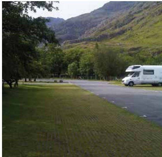
Figure 20.5 Concrete grids in a park and ride overflow car park, Gwynedd (courtesy EPG Limited)
