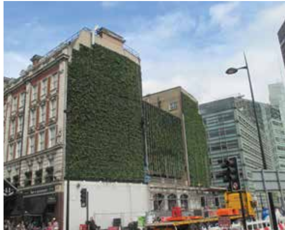
Green wall (courtesy Green Roof Consultancy)
