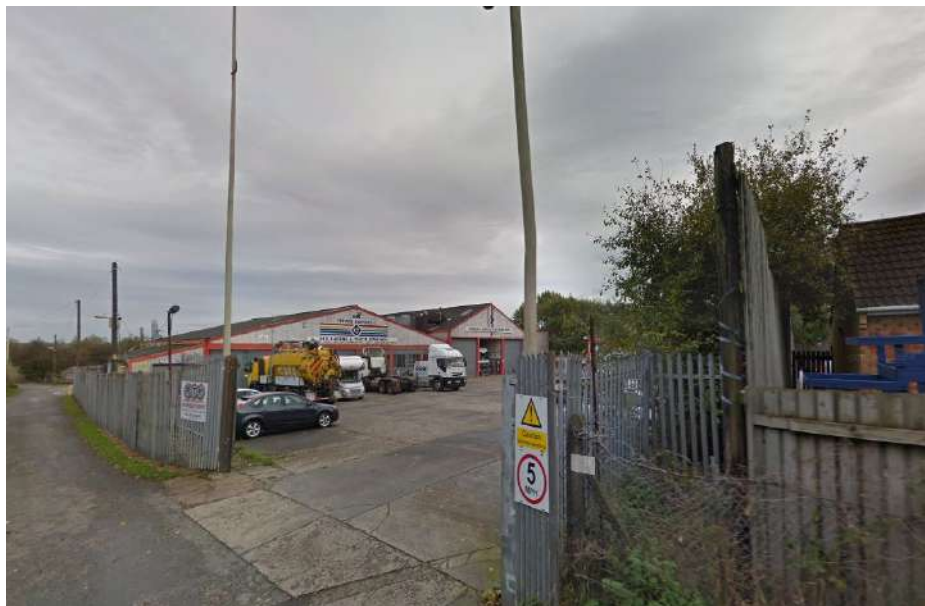
Fig. 15 View - 4 Existing industrial site (North-East)
