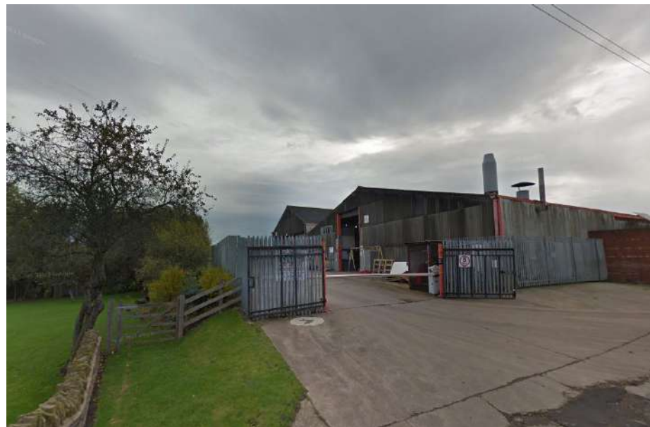
Fig. 16 View 5 - Existing industrial site (North-East)
