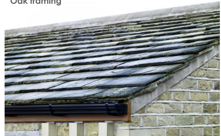
Reclaimed natural Yorkstone roof slates, laid in diminishing courses
