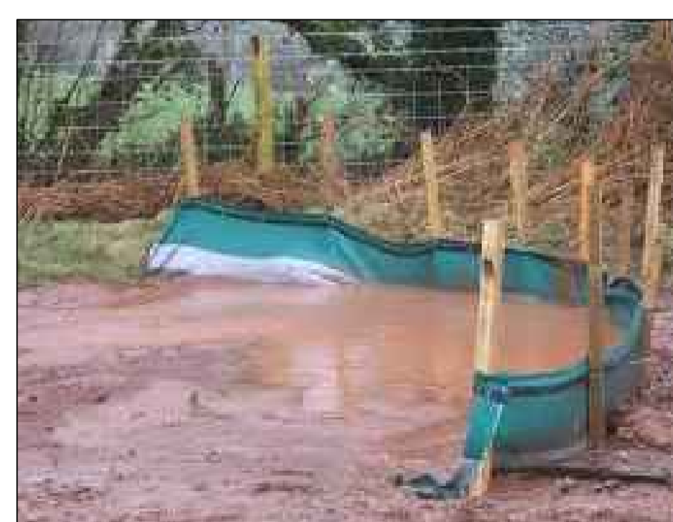
DIRTBAGS SEDIMENT CONTROL PRODUCT OR SIMILAR (REFER TO MANUFACTURERS INSTALLATION GUIDANCE)
