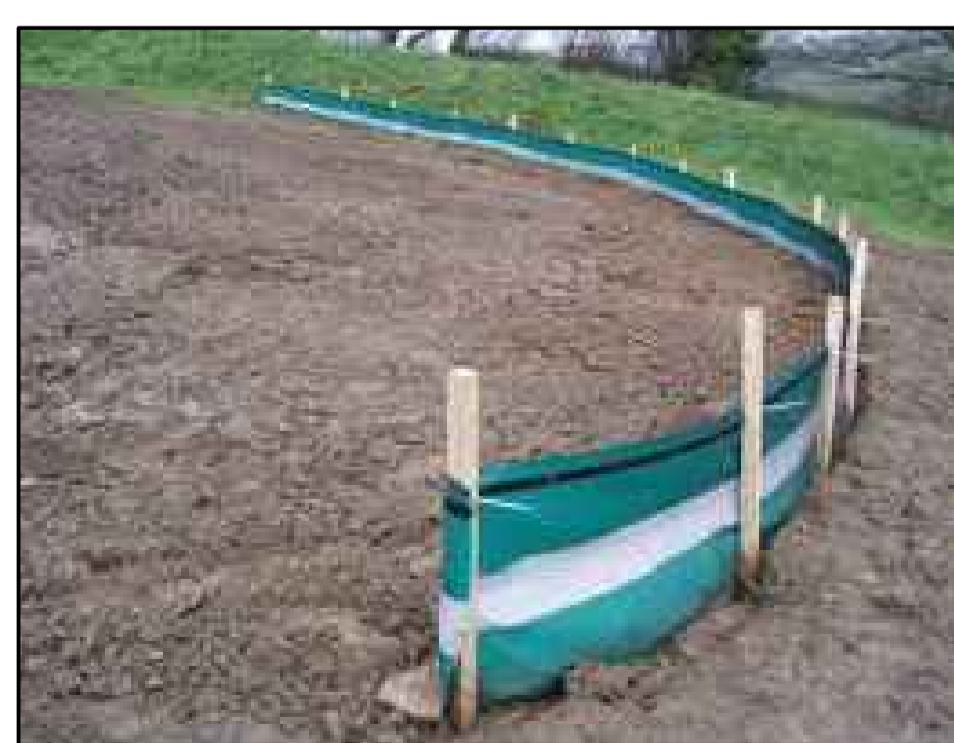
DIRTBAGS SEDIMENT CONTROL PRODUCT OR SIMILAR (REFER TO MANUFACTURERS INSTALLATION GUIDANCE)
