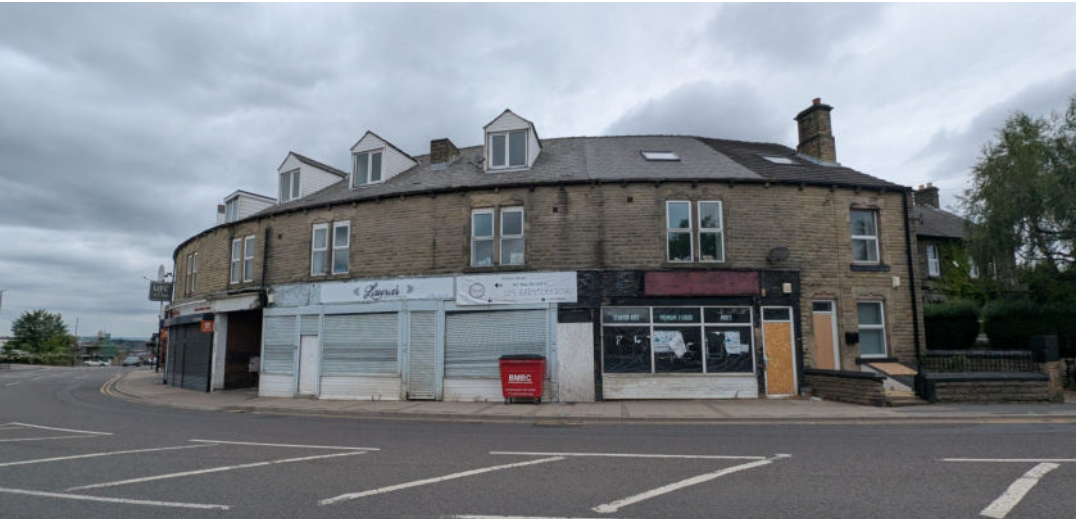
1. View of the existing buildings on site, looking South West.
