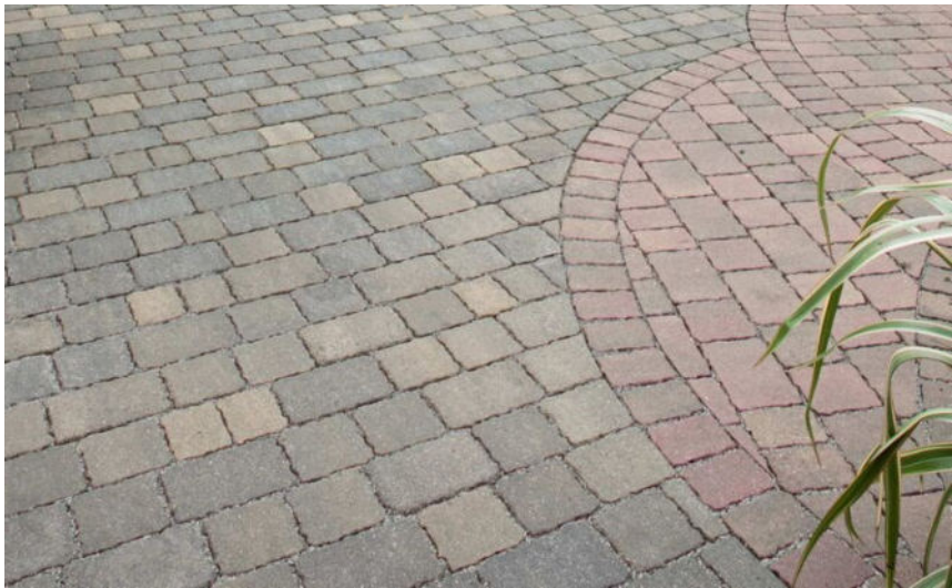
4. Concrete pavers in contrasting colours, arranged in various patterns.
