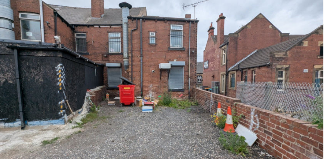
3. View of the rear of the existing buildings.
