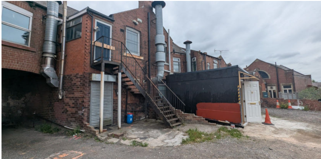
1. View of the existing buildings at the back. Multiple commercial flues, external stairs, blocked up doors and windows.
