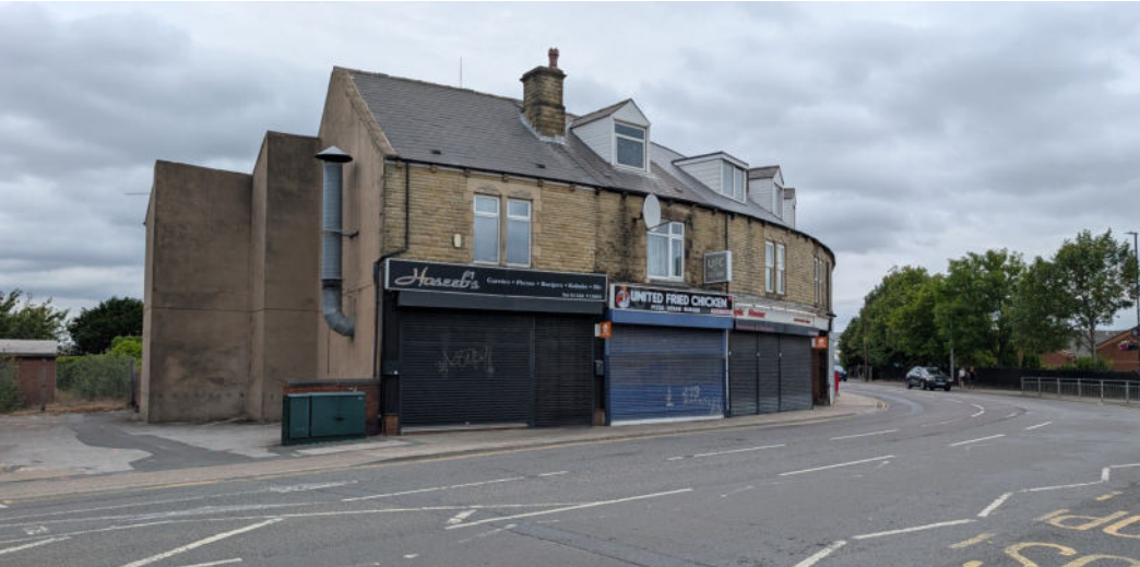
2. View of the existing buildings on site, looking North East.
