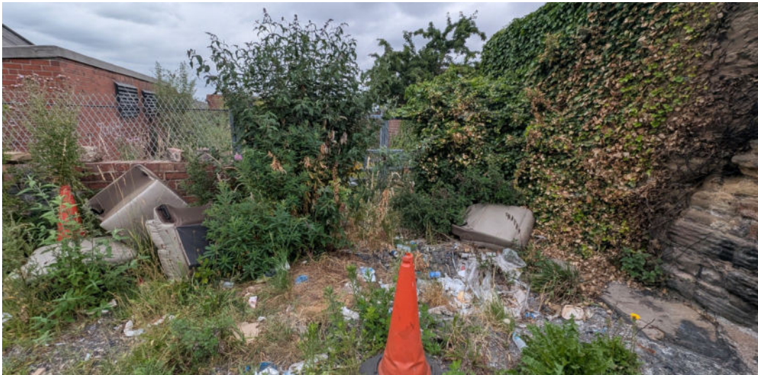
2. Part of the site being vandalized, used for fly tipping and other anti-social behaviour.
