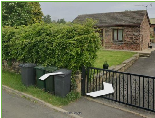
Front Elevation of the Existing Bungalow. [source: Google Streetview]
