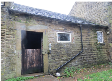
Photo 02 - Front view of Workshop
