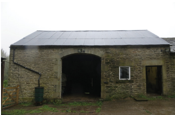
Photo 01 - Front view of Barn
