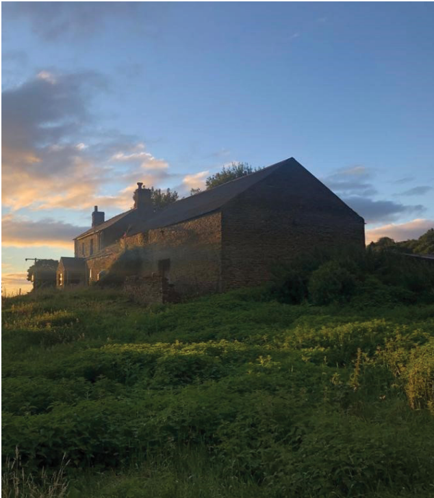
Existing photo looking at rear of farm-house & barn
