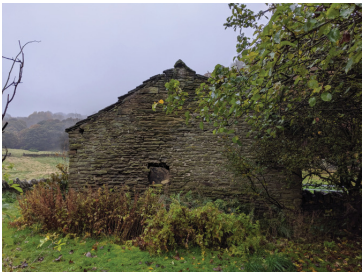
Photo 07 - Side View of Slaughter House
