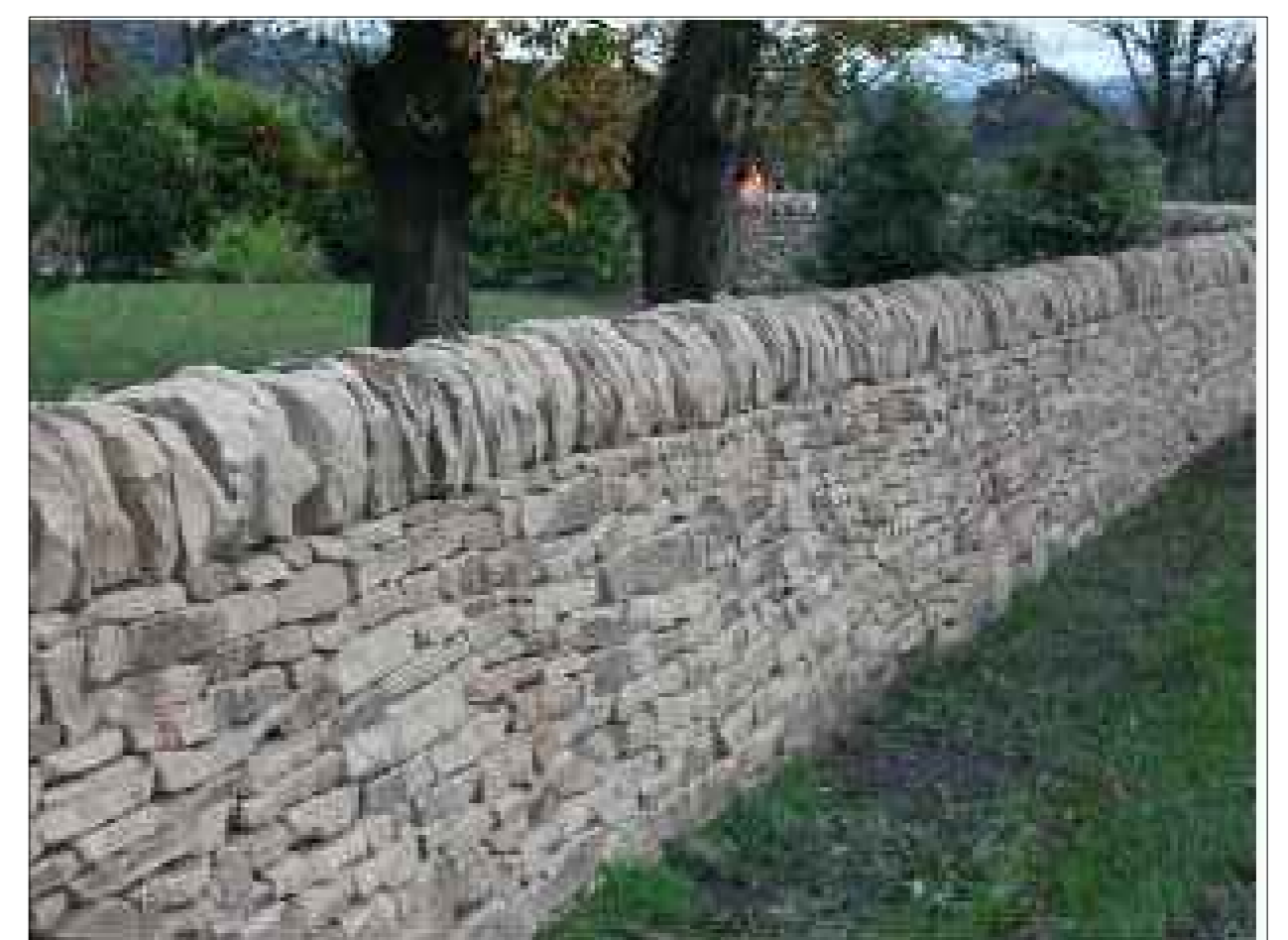
Dry stone walling feature to entrance bellmouths. (behind Visibility Splays) approx 1500 high approx 20m length (each) built using local / reclaimed stone by a Local Stonemason
