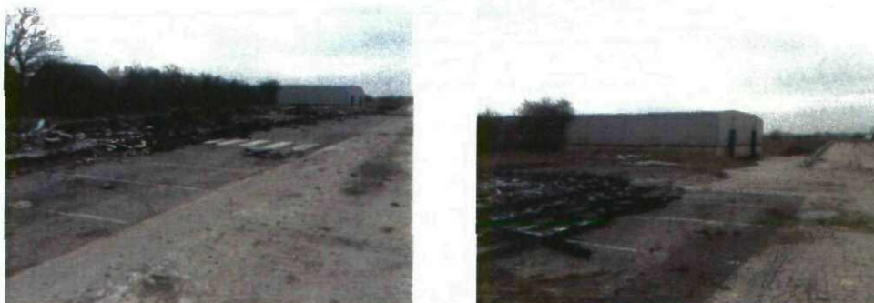
Figure 2.3 – Location of fire damaged / destroyed timber framed building
