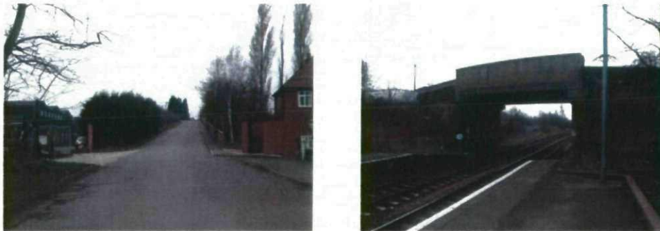
Figure 2.1 – Access to the subject site from Lowfields Road and the Railway Bridge
