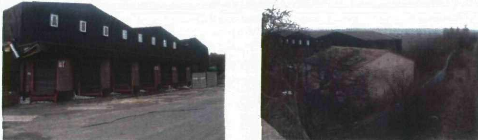
Figure 2.2 – Extension block to west of North Light Block
