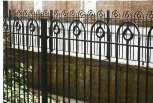
Harriseahead bow top railings
