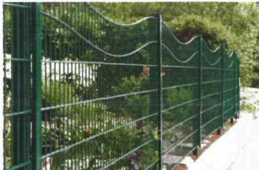
Wavetop security fencing
