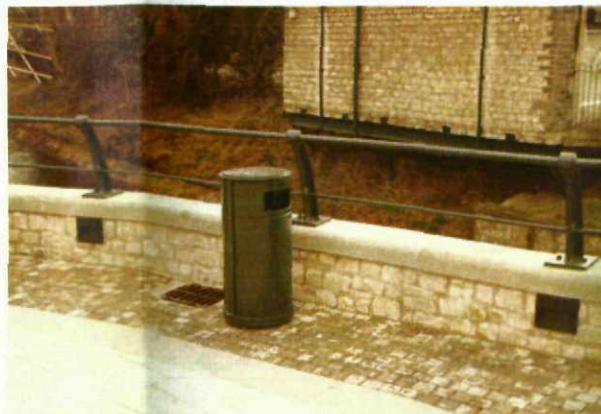
Quayside guard rail
