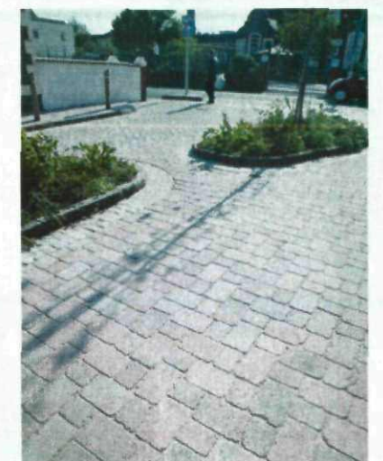
Tegula Traditional block paving
