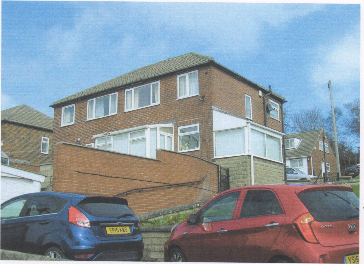
STAIR REAR / SIDE
