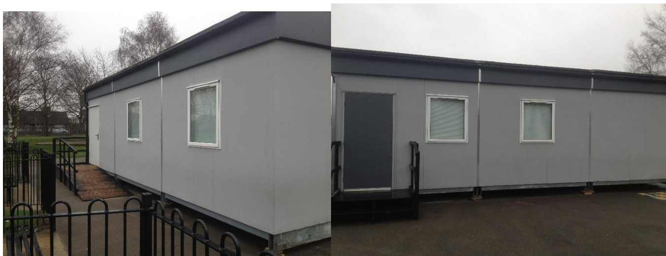
Declared Temporary Cabin Classroom on site.
