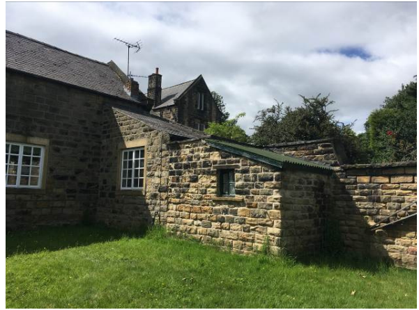
Fig 11 Single storey rear extension and outside toilet
