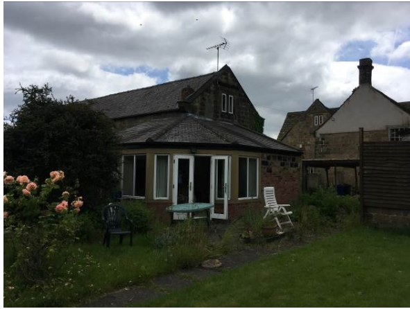
Fig 10 Single storey rear/side extension
