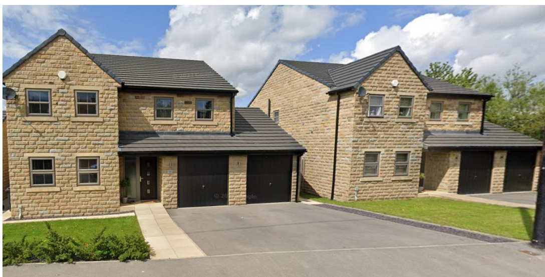
Photo 5.1: Recently Constructed Housing Nearby
