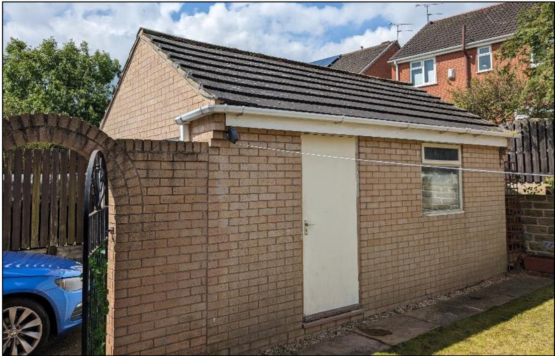
Plate 8. Well pointed verge on east gable of garage
