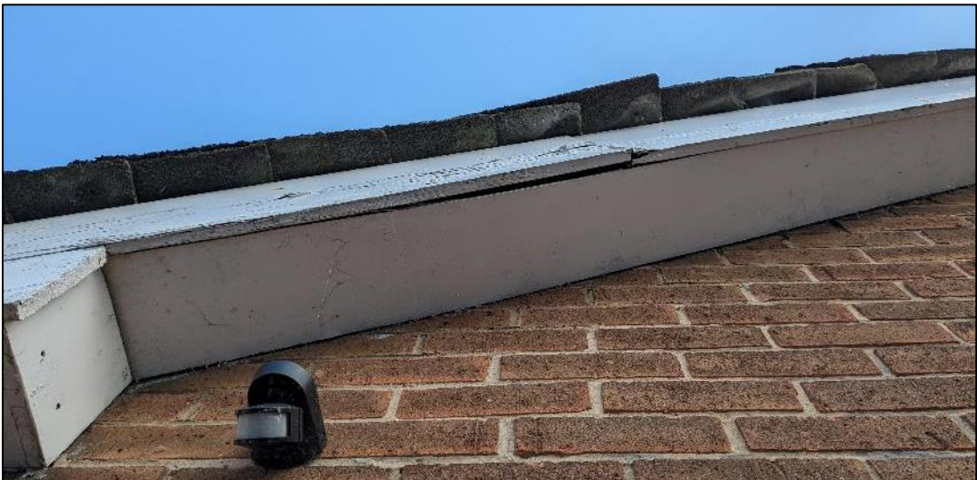
Plate 4. Faulty barge board on south gable
