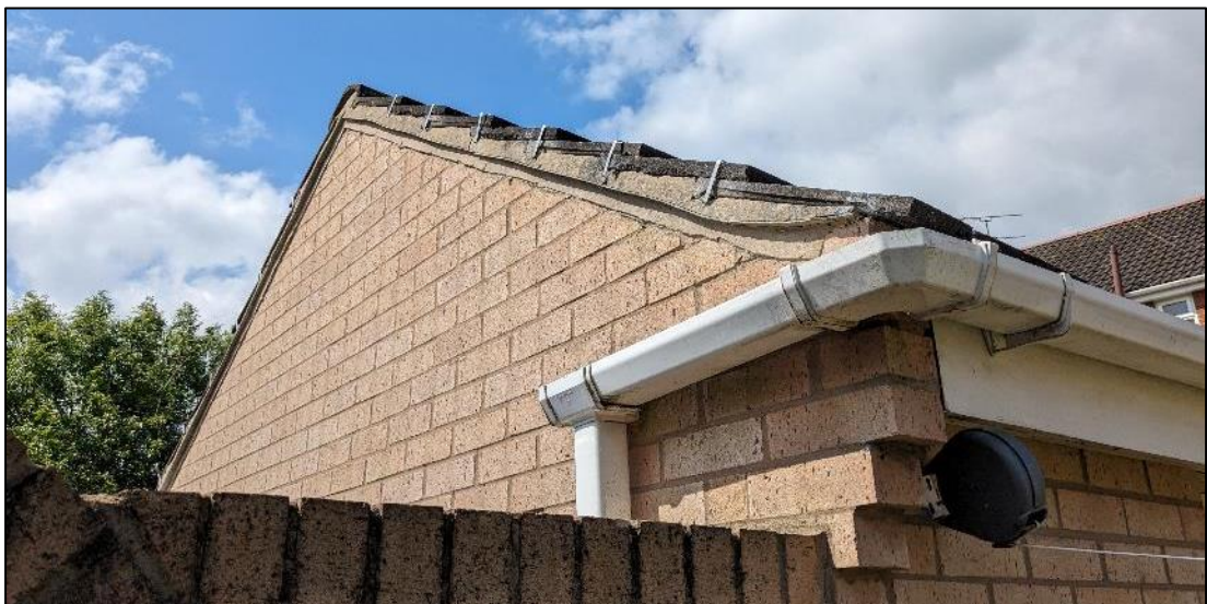
Plate 8. Well pointed verge on east gable of garage
