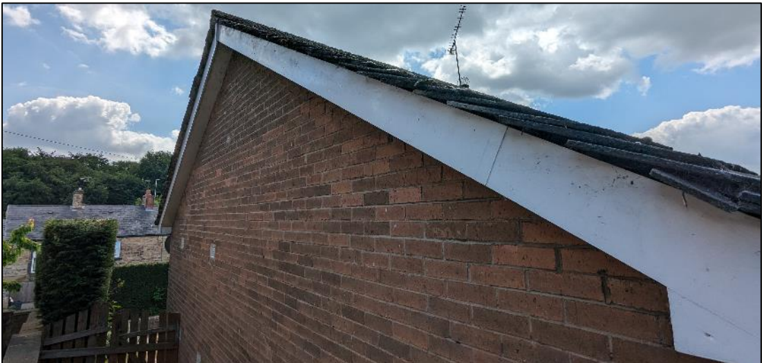
Plate 4. Faulty barge board on south gable
