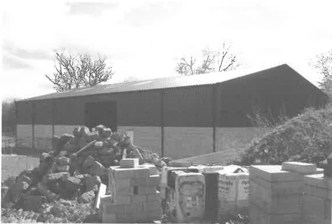
View of Existing Building with Storage Area in Front
