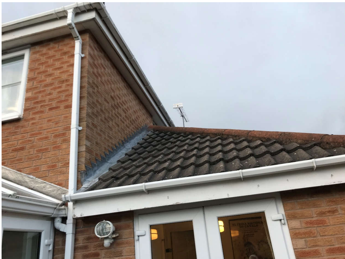
06. Rear south east corner.
