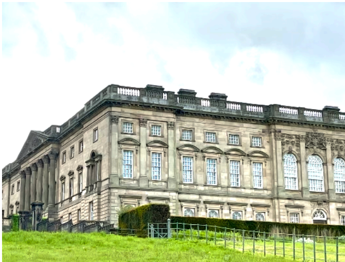
The base of the chimneys and the antenna are screened by the parapet walls.
