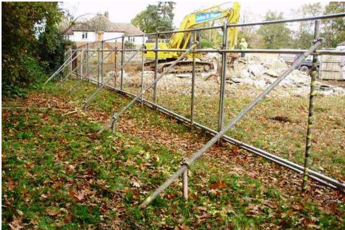
Figure 2: Photo of Fencing to BS 5837: 2012
