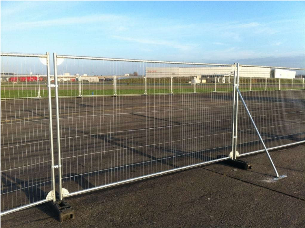
Figure 5: Secured 'Heras' type fencing with stabilizing system and anti-tamper couplers
