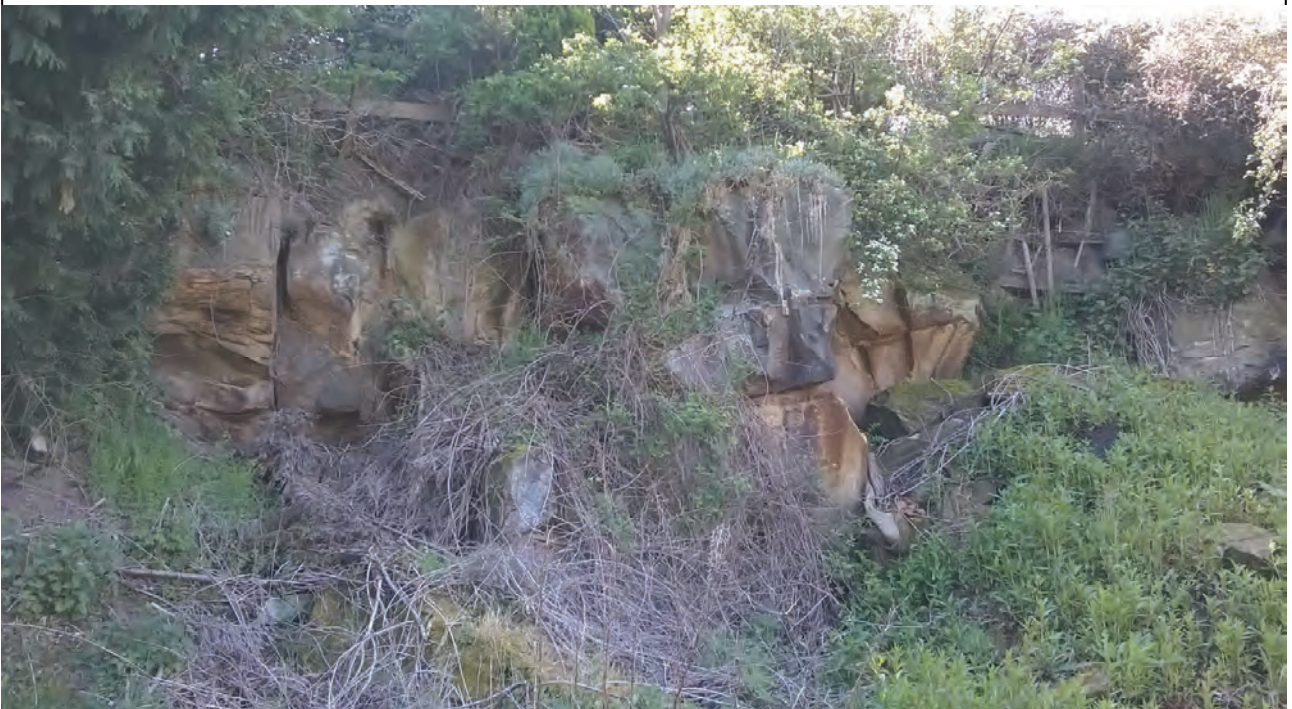
Photo 2 : Looking at rock face which forms southern boundary. Loose blocks noted.
