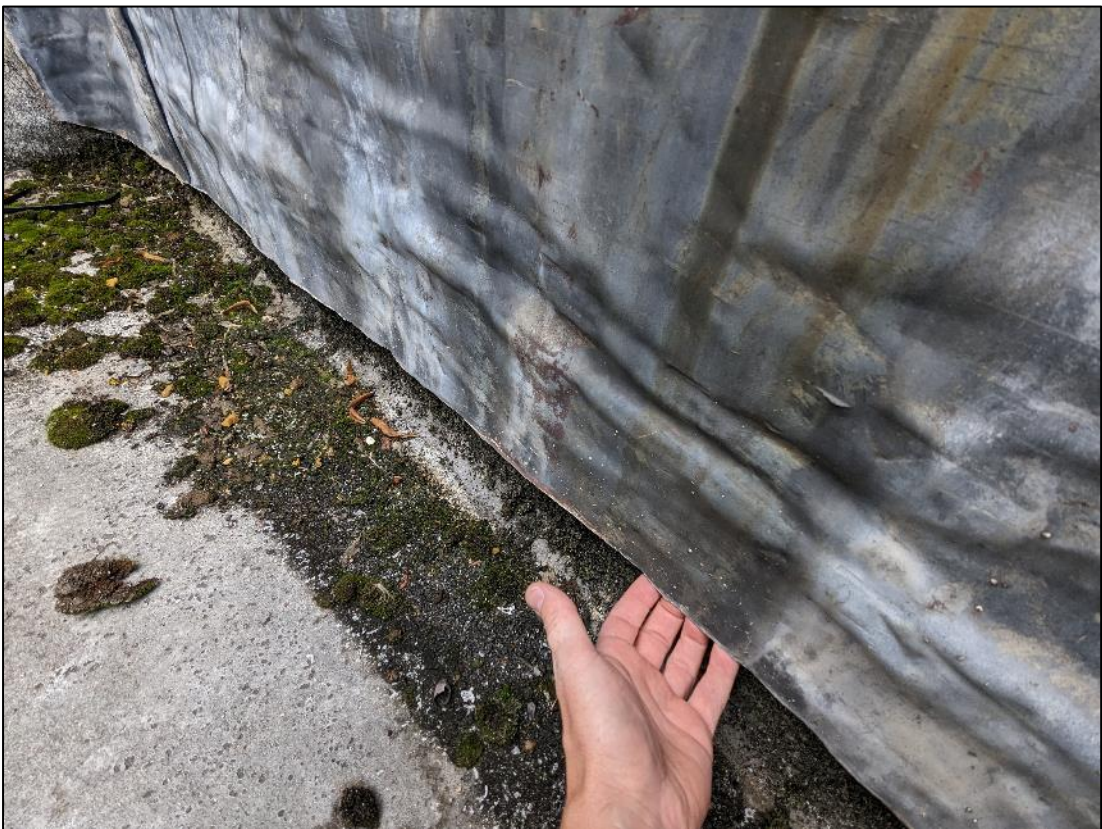
Plate 8. Section of lifted flashing on internal face of parapet
