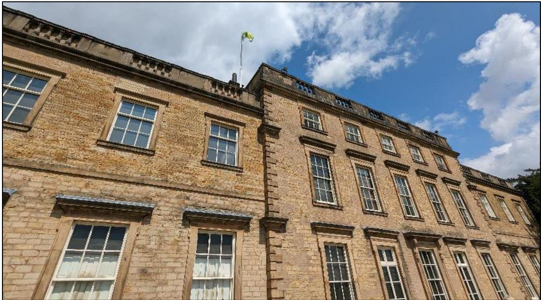
Plate 1. Southeast elevation of Cannon Hall
