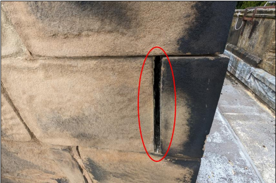
Plate 8. Section of lifted flashing on internal face of parapet
