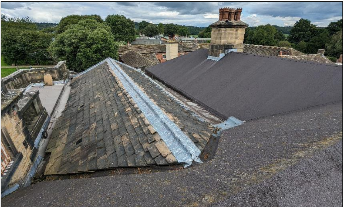
Plate 6. Kitchen roof, including small section of stone slate covered roof
