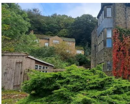
Fig 15 New dwelling above Parsonage House
