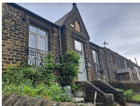
Fig 12 Former Methodist Chapel, now dwelling, much altered to accommodate conversion
