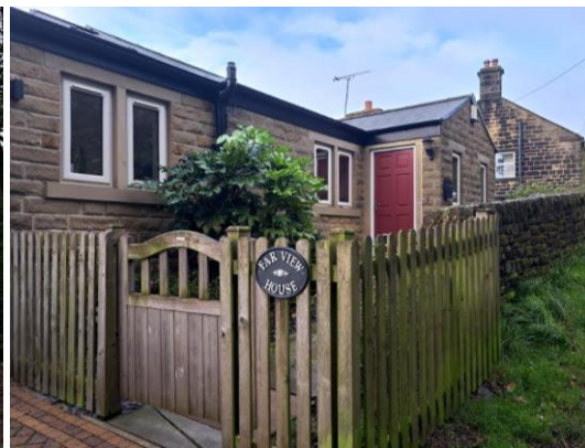
Fig 63 Far View House fencing and mullions
