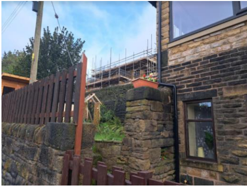
Fig 60 House above High Bank Lane
