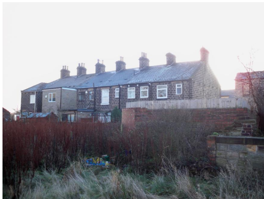
Rear of Terraced Properties to High Street to the South of the Site
