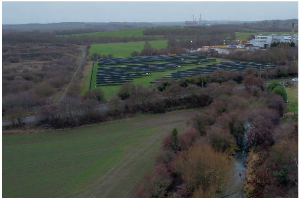
Figure 10 - view onto south of Shaw Lane
