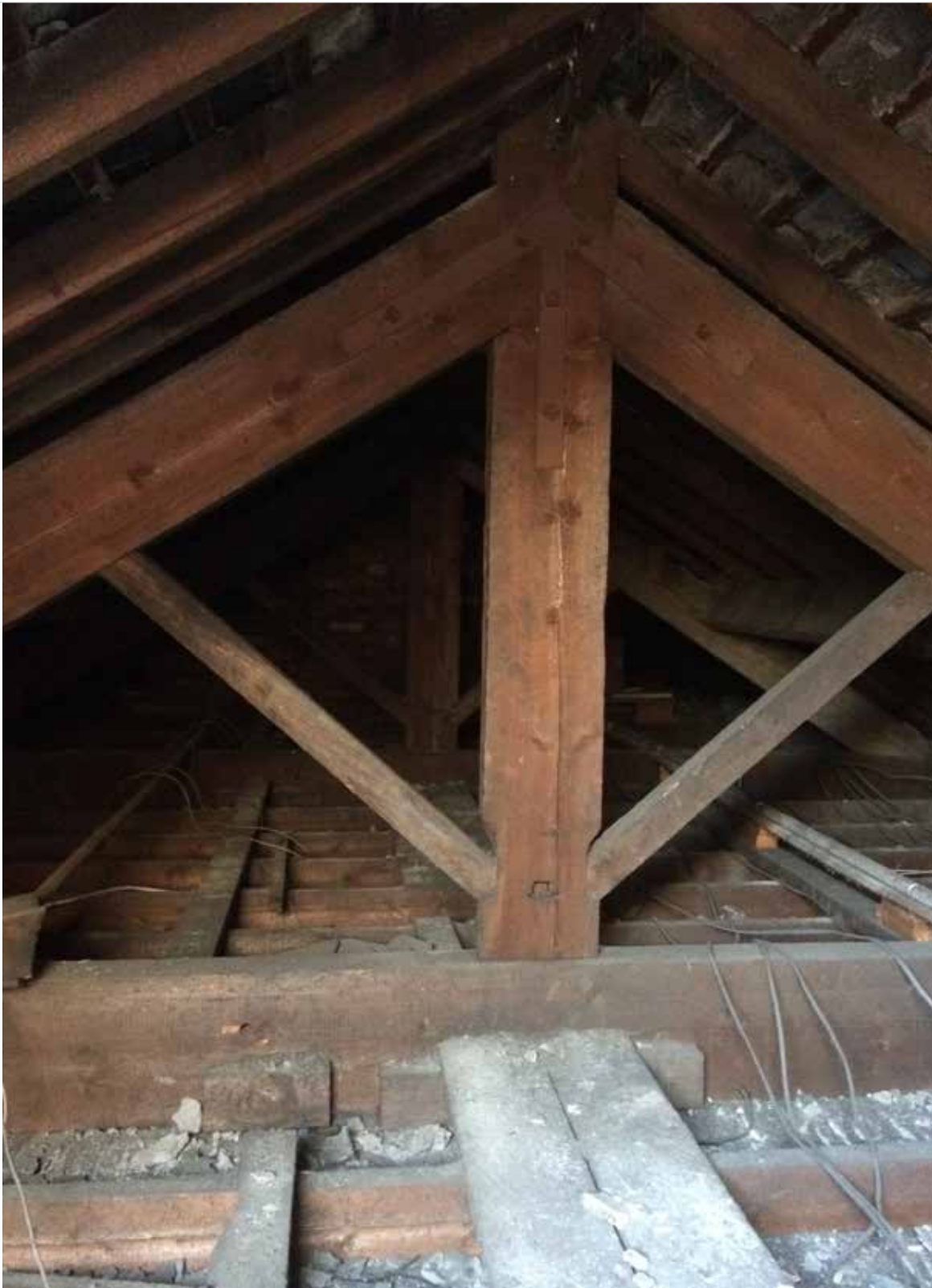
Existing Roof Structure
