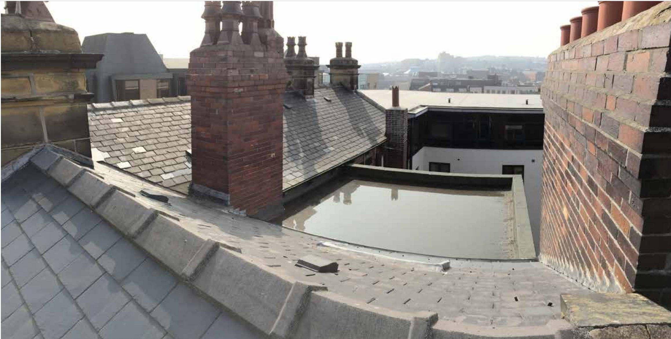
Existing Roof Looking into Courtyard
