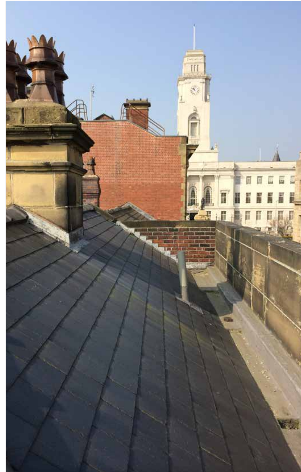
Existing Roof Looking West
