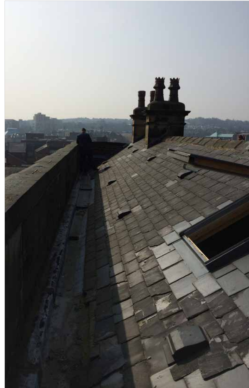
Existing Roof Looking South
