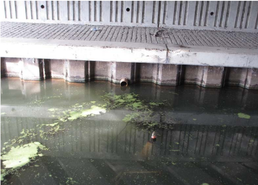
End of Highway drain into canal below A6195 approximately 200m south of site. Assumed To drain part of carriageway.
