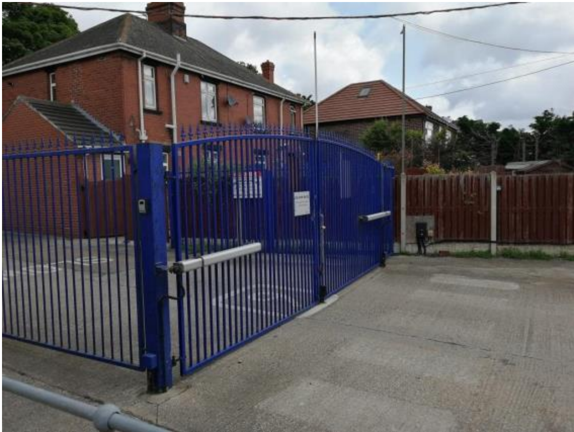
Photograph 3: Security gates at site entrance
