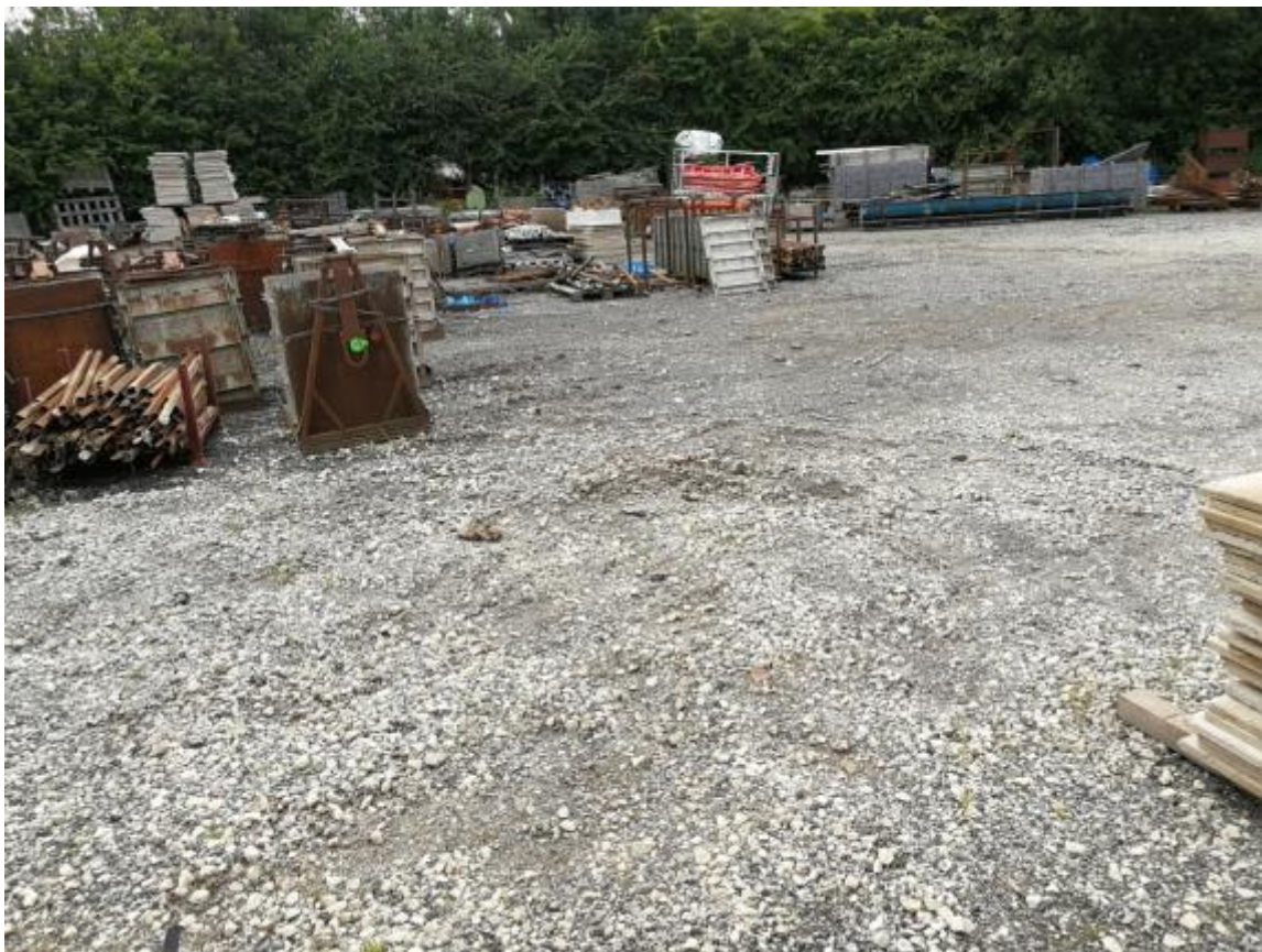
Photograph 22: Hardcore area at far south of site used for storage of equipment
