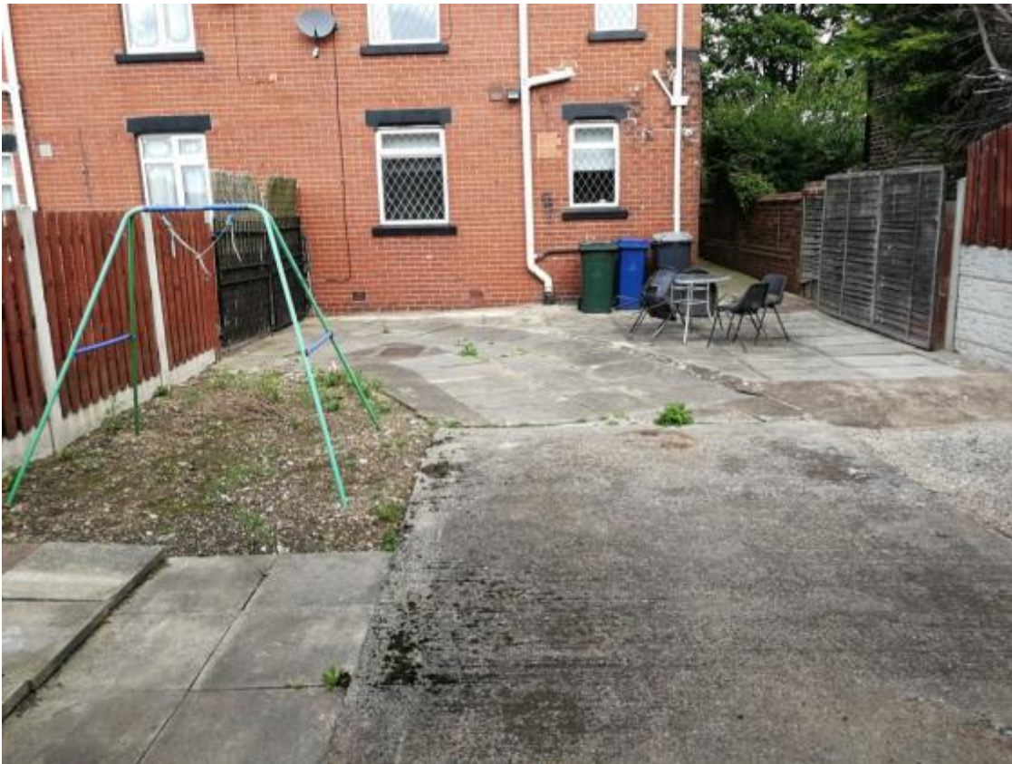
Photograph 49: Semi detached houses on Hough Lane adjacent to site offices. Houses owned and used by Balmoral tanks.
