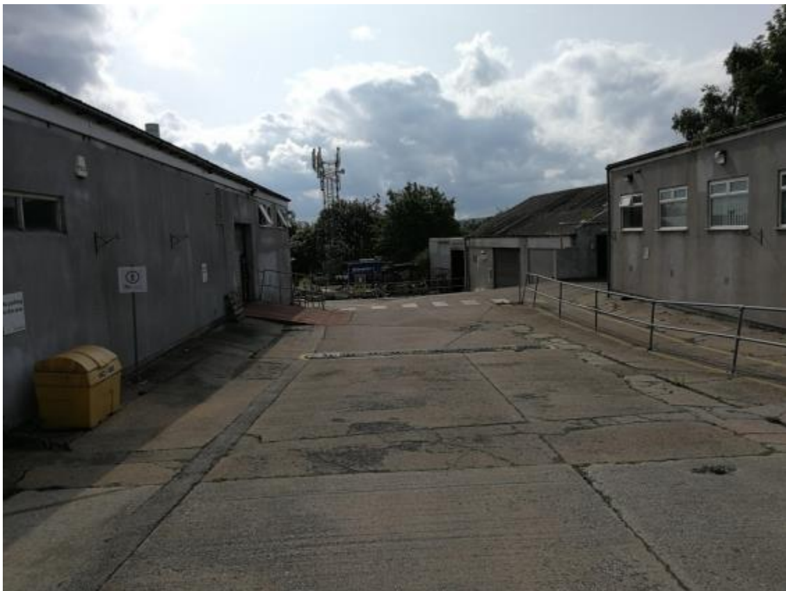
Photograph 6: Epoxy spray painting workshop to the left, office building to the right, maintenance workshop to the far right and telephone mast in the distance.
