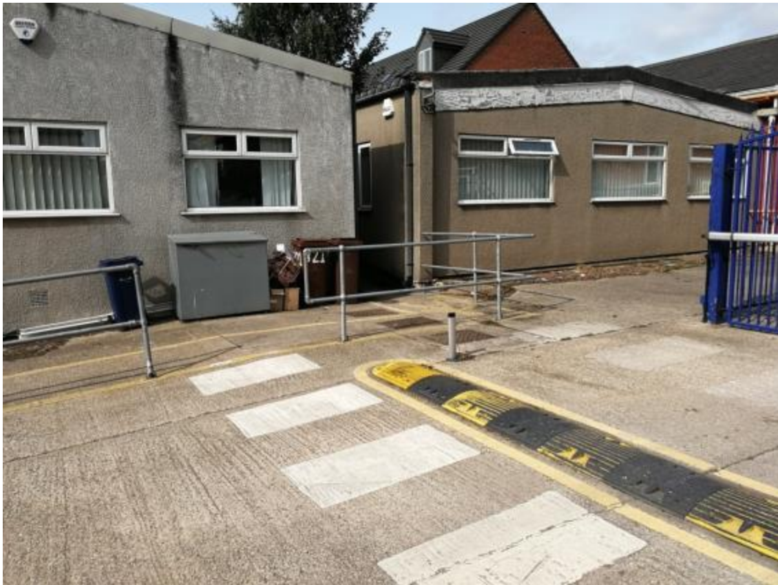
Photograph 5: Office buildings in the north west of site
