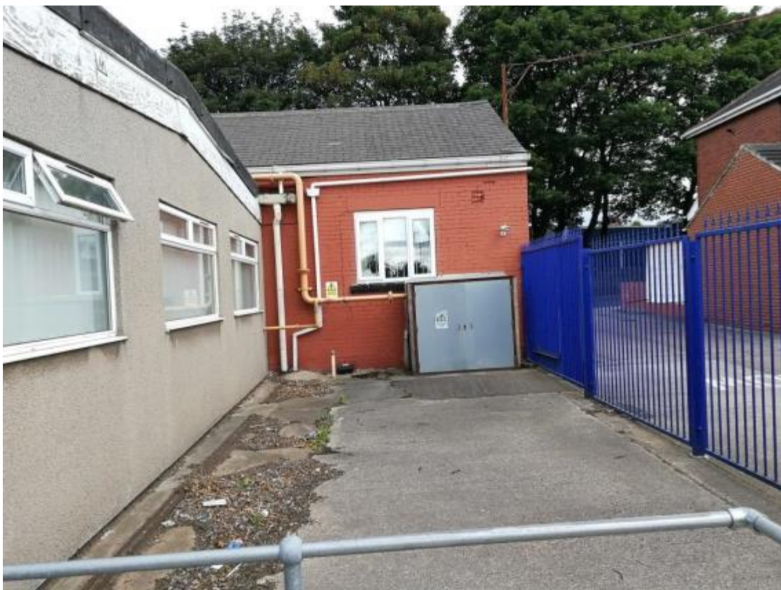
Photograph 4: Gas main connection
