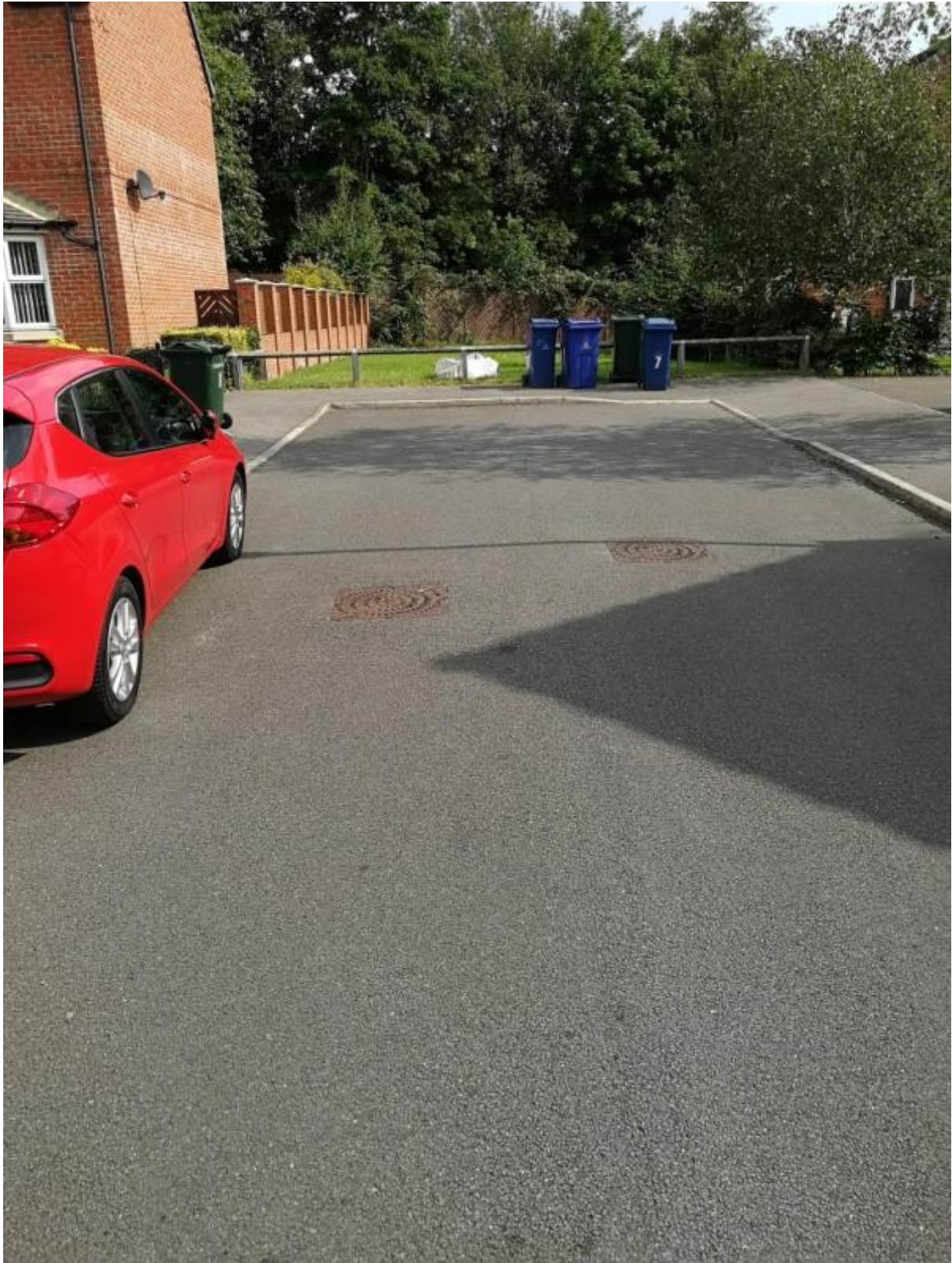
Photograph 50: Manhole covers on Malsin Gardens.
