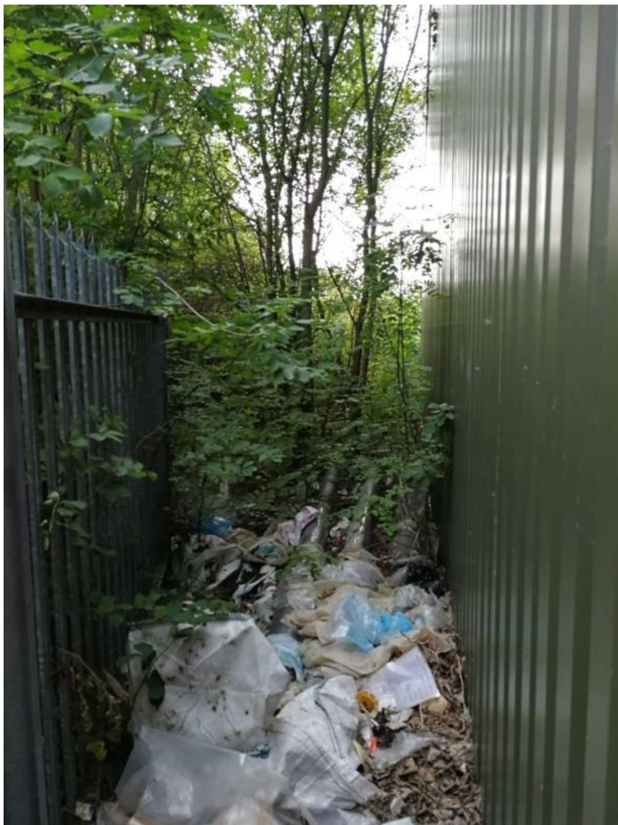
Photograph 37: Eastern extent of the site, between the boundary fence and the workshop.
