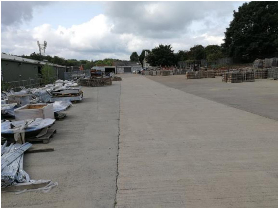
Photograph 39: Concrete hardstanding in front of welding and fabrication workshop
