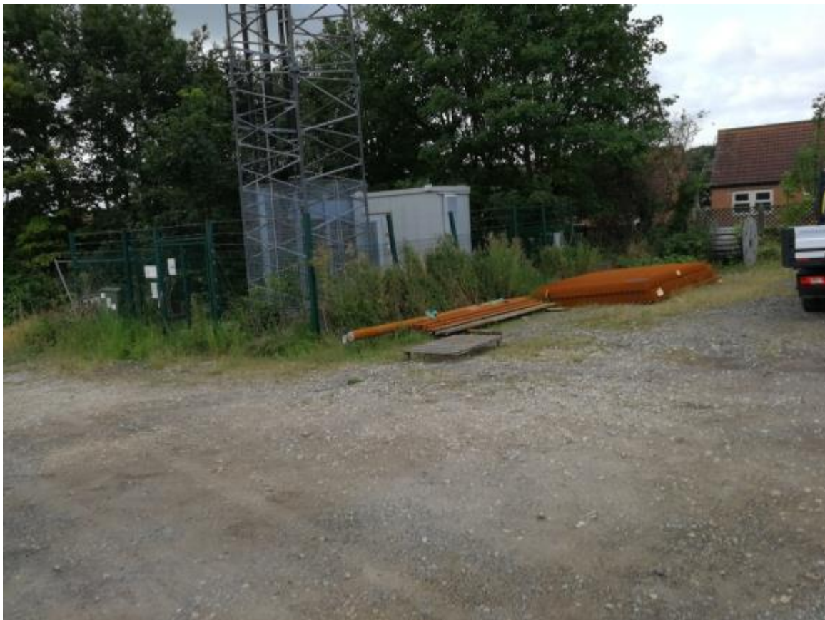
Photograph 18: Mobile phone mast compound
