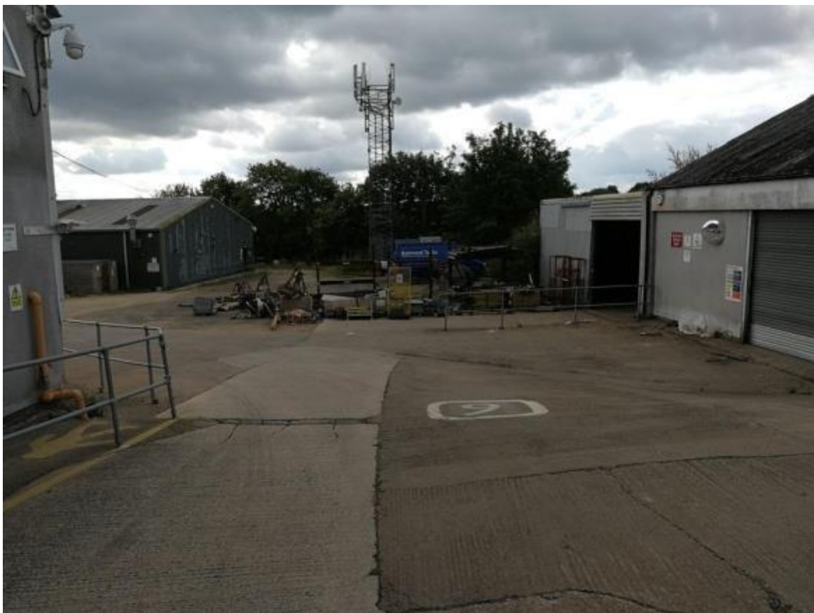
Photograph 10: Maintenance workshop to the right
