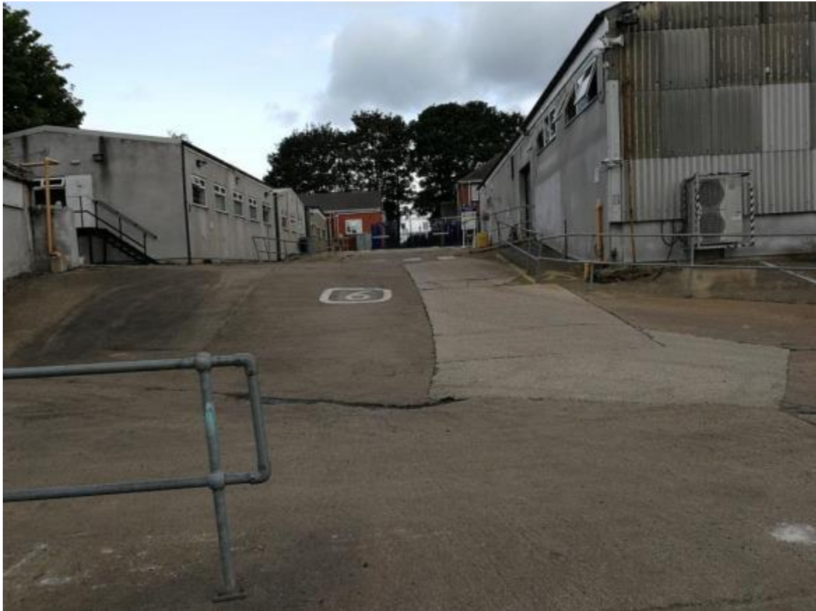
Photograph 15: View up towards site entrance
