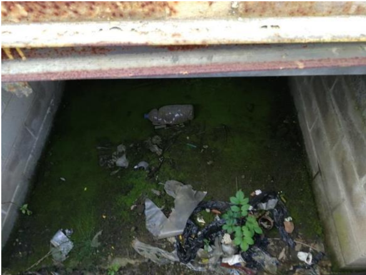
Photograph 35: View beneath the tank
