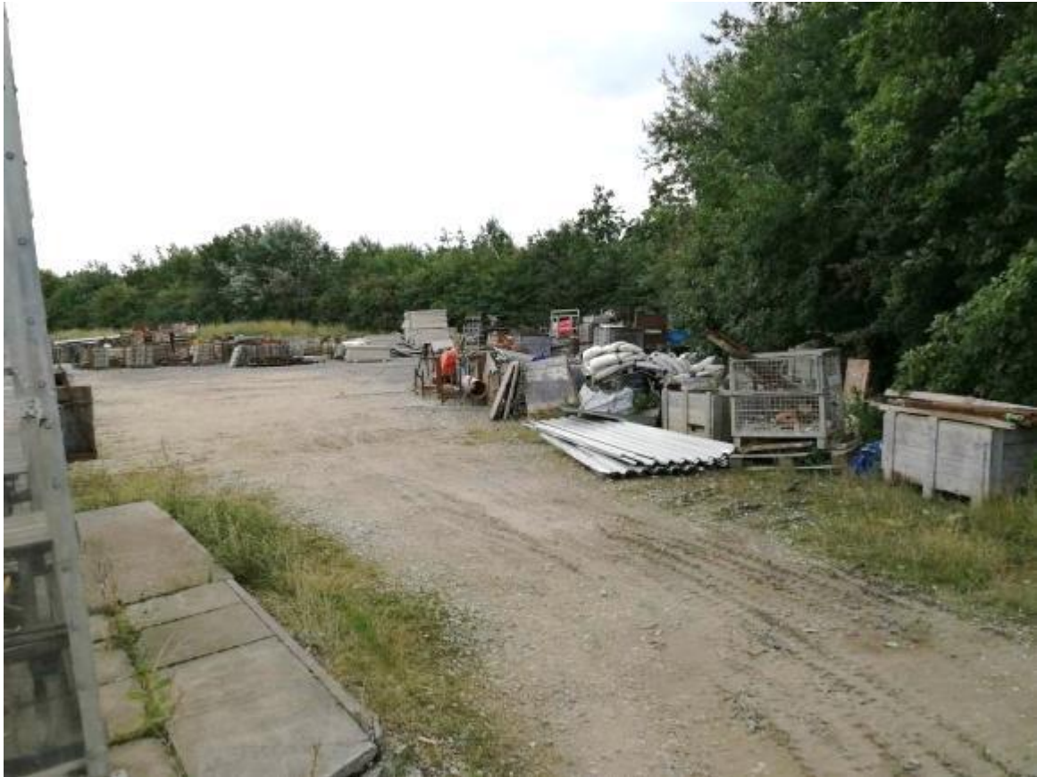
Photograph 21: Hardcore area at far south of site used for storage of equipment
