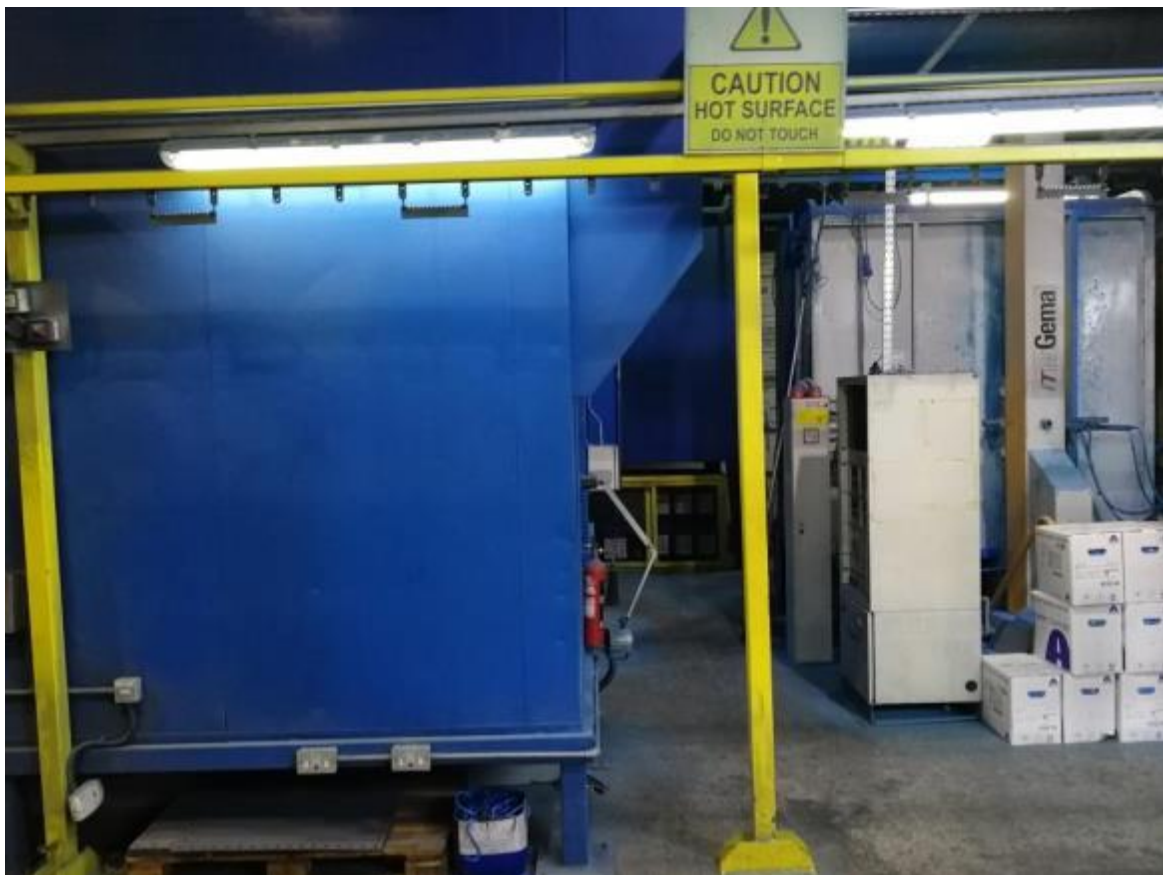
Photograph 8: Interior of spray painting workshop
