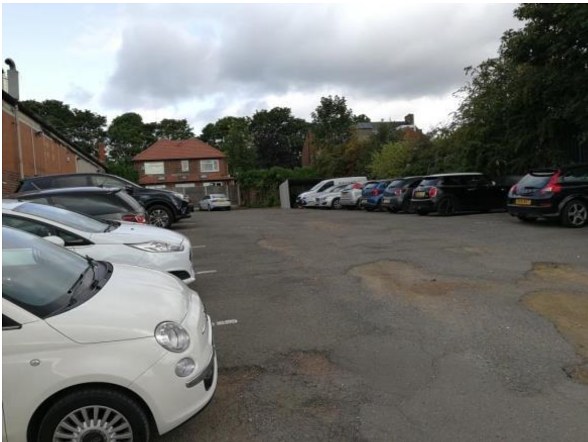
Photograph 16: Car park to the east of the spray paint workshop
