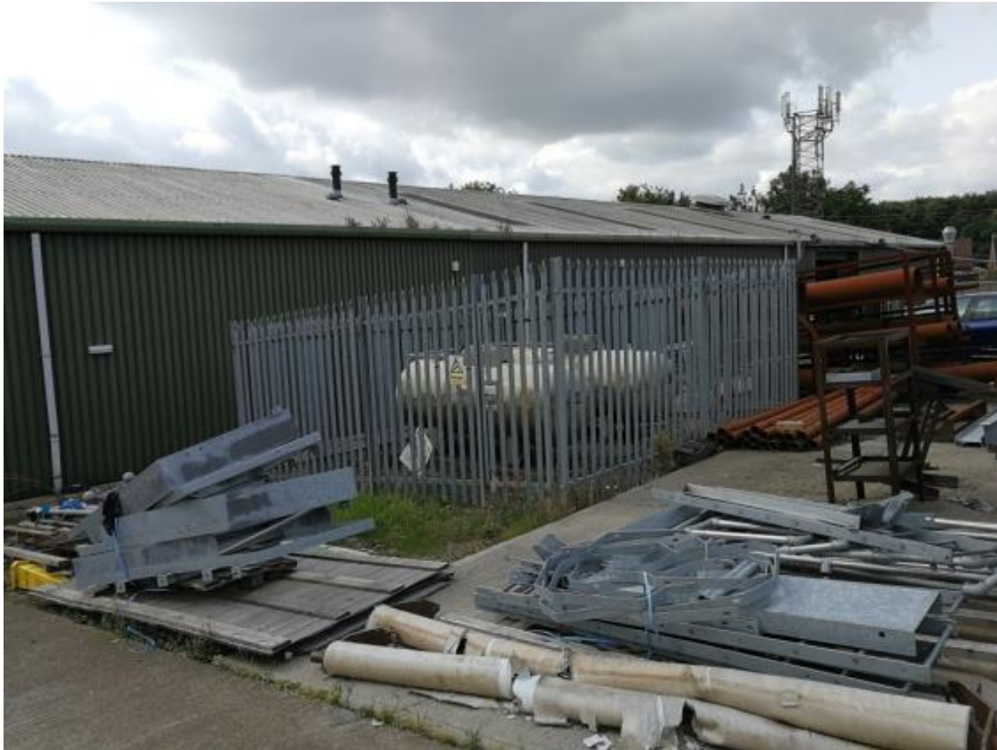
Photograph 42: 2 No above ground propane gas tanks within secure compound
