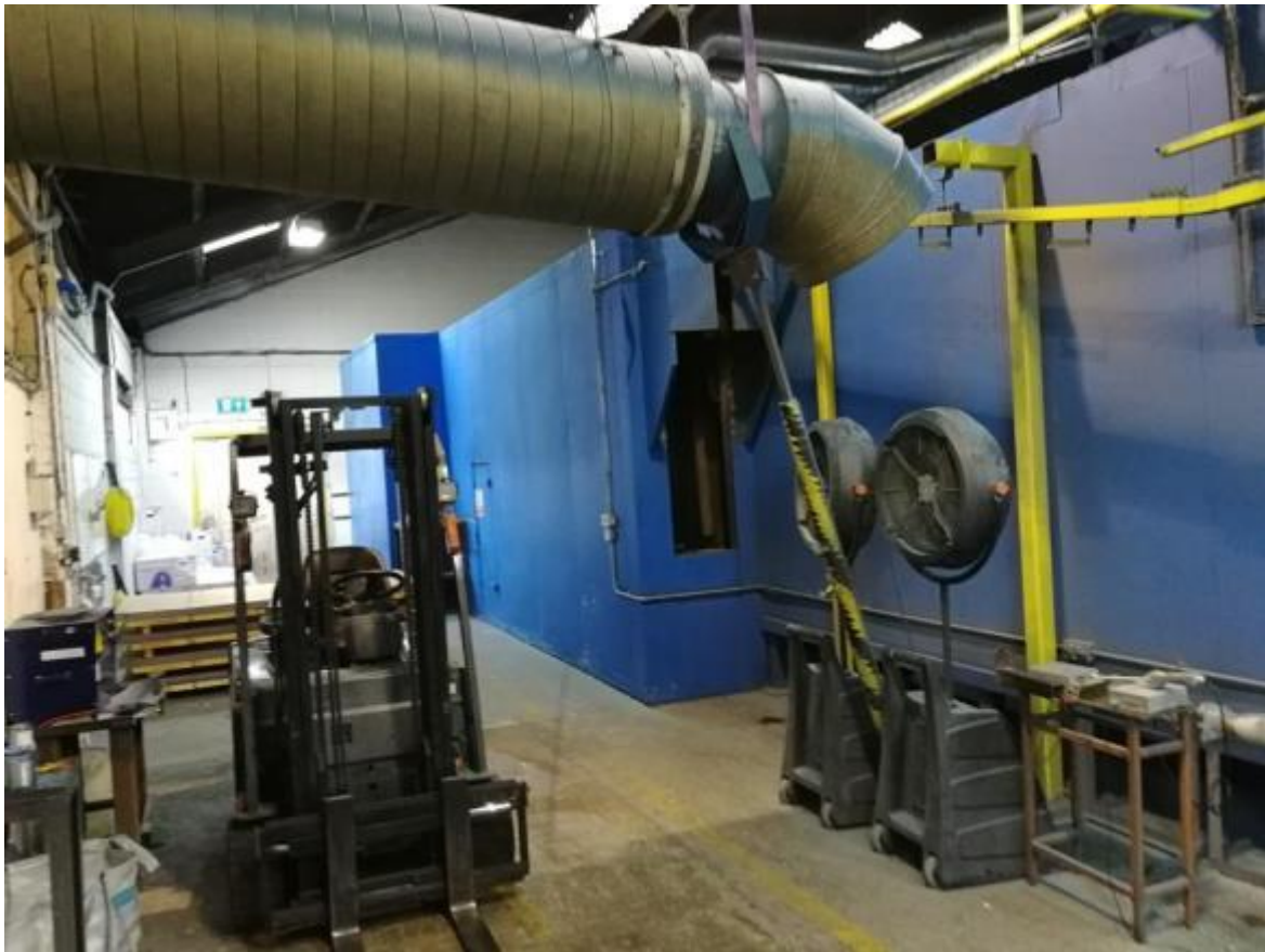
Photograph 9: Interior to spray painting workshop
