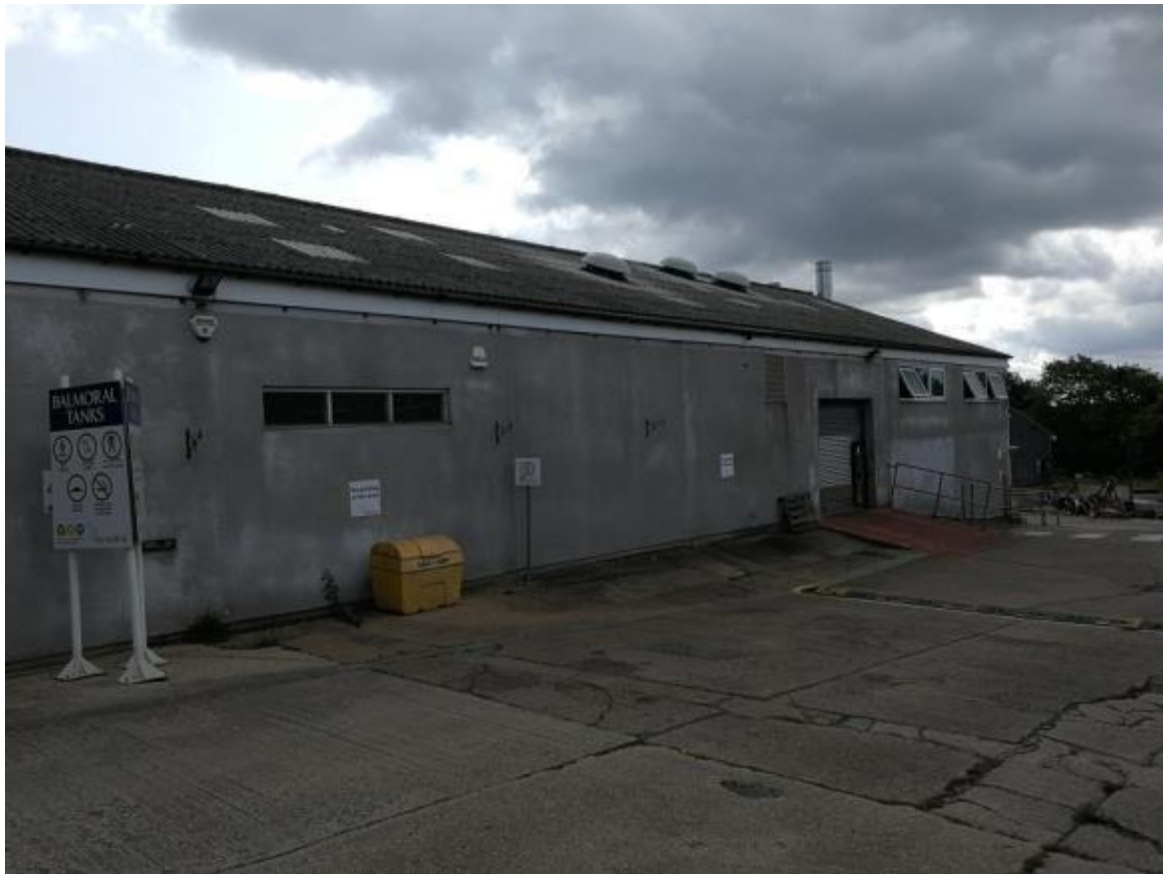
Photograph 7: Epoxy spray painting workshop
