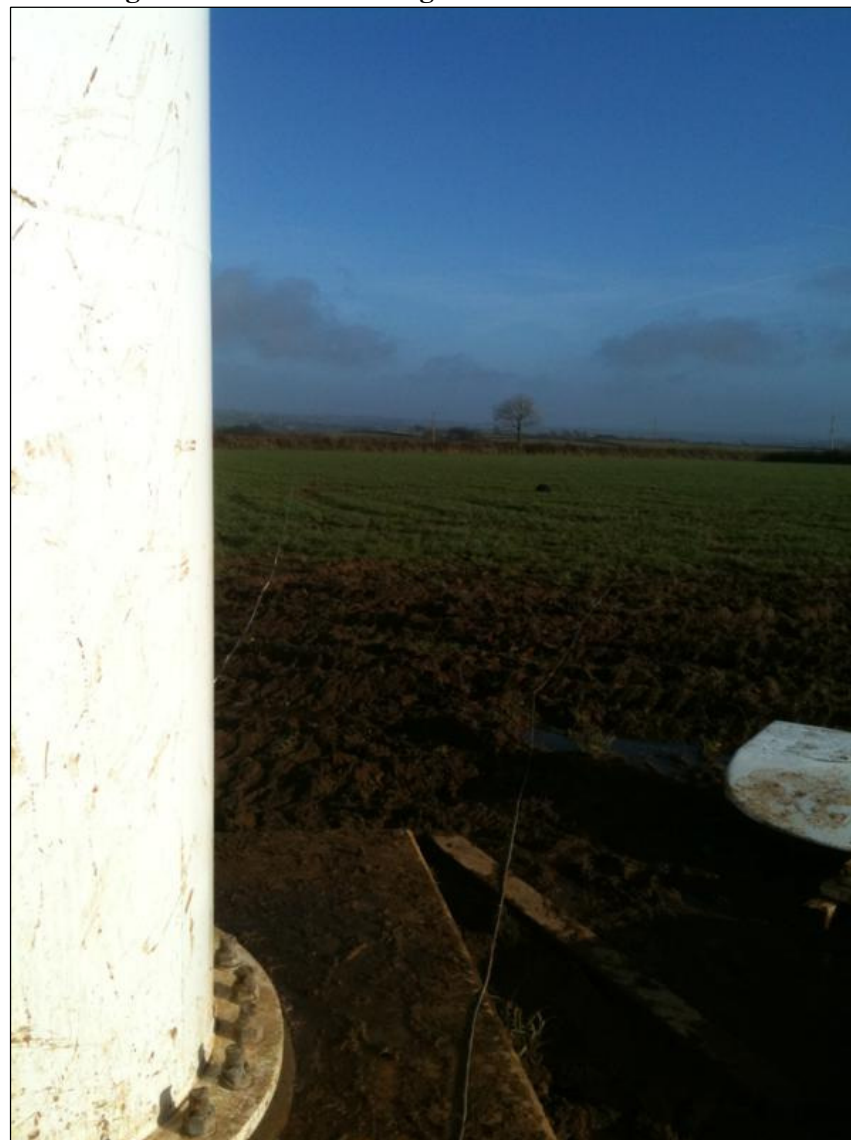
Figure B2 –Photo Showing View of Ground Board from Turbine
