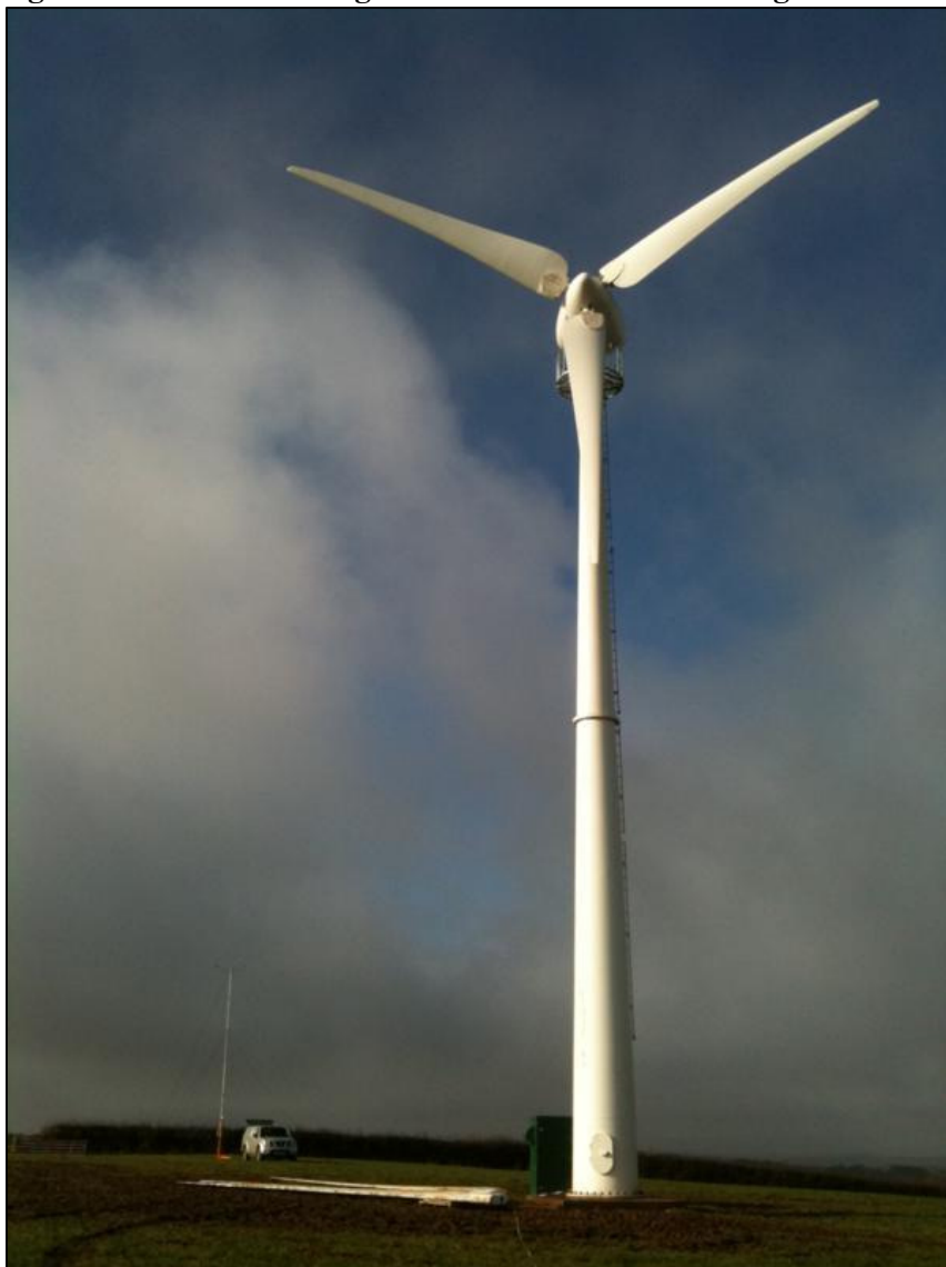
Figure B1 –Photo Showing Turbine and 10m Meteorological Mast
