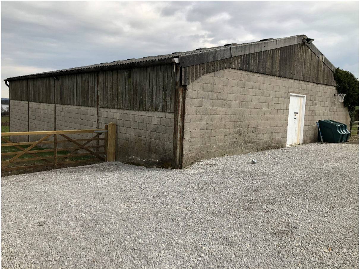
Existing building to be removed
