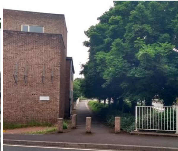
Rear elevation to Westway screened by trees
