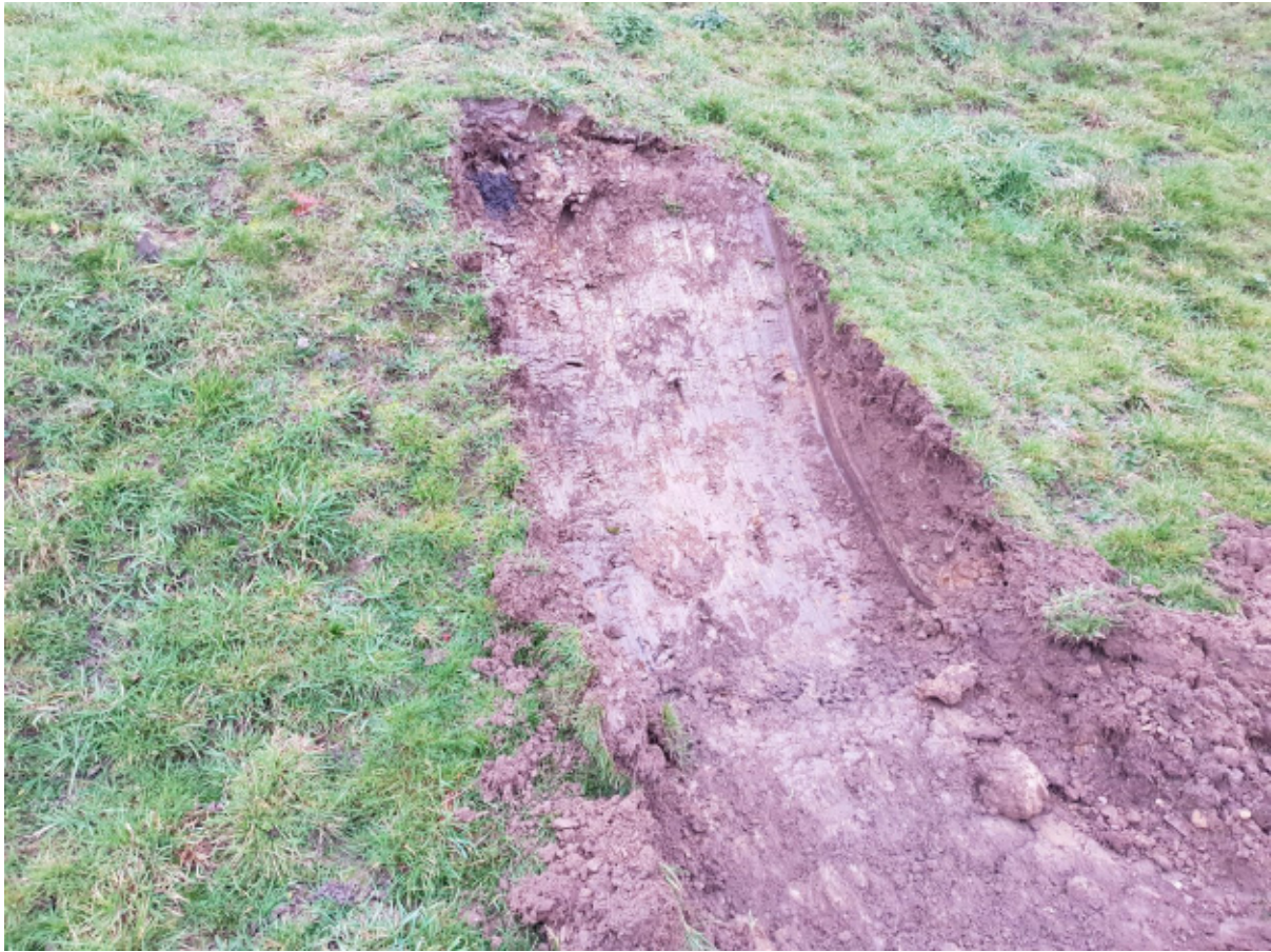
Shallow excavation in to earth mound in north east
